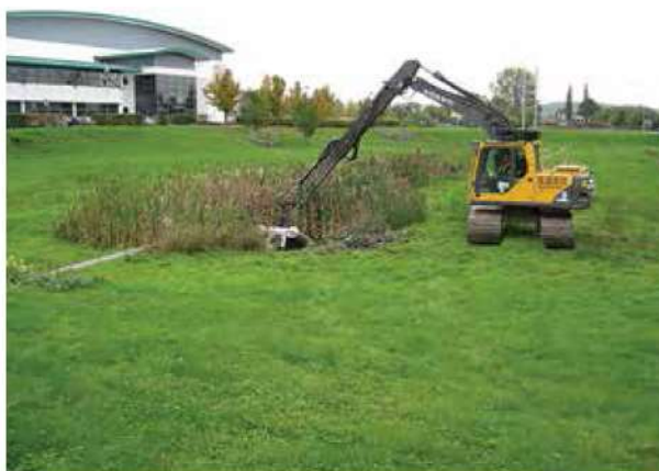
Figure 32.2 De-silting (courtesy Bedford Group of Drainage Boards)
