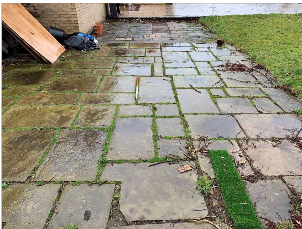
Photograph 9: View of possible original flagged area.
