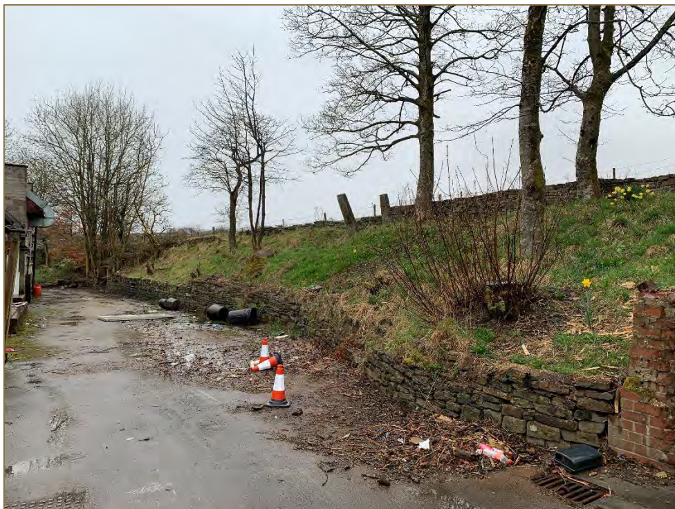
Photograph 6: View east over the PDA, dry stone wall embankment
