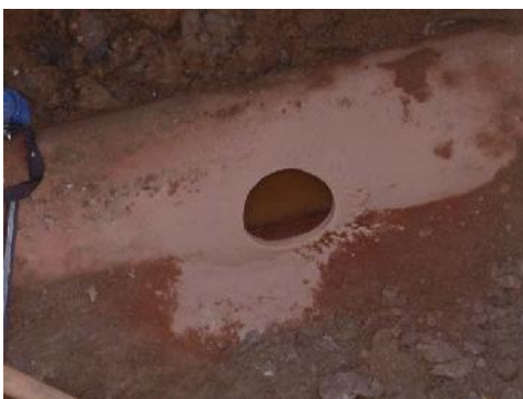
Hole core drilled ready for saddle
