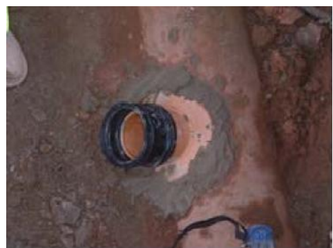
Saddle in Place
