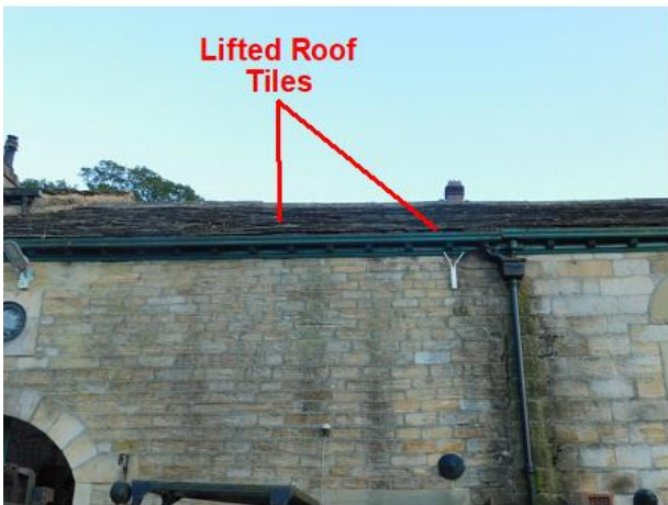
PHOTO 21 Western Roof Edge
