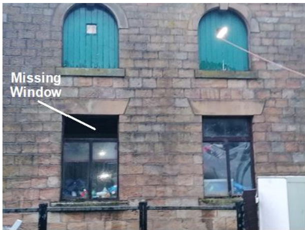
PHOTO 7 View of Western Wall
