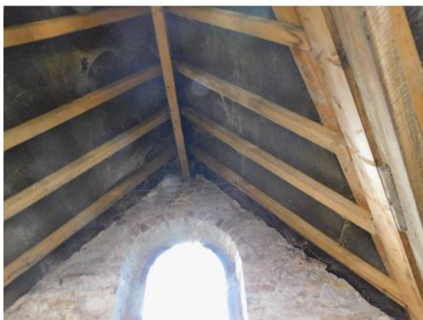
PHOTO 27 Underside of Northern Dormer Roof
