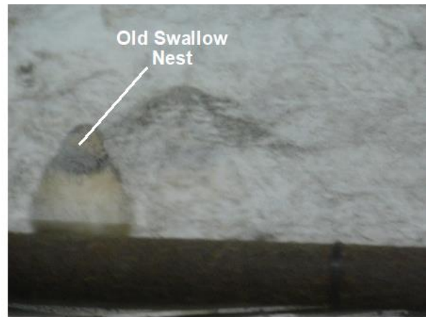
PHOTO 36 Upper Internal Eastern Roof
