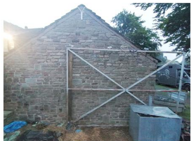
PHOTO 12 Northern Elevation of Henhouse
