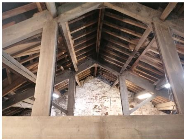
PHOTO 26 Underside of Eastern Roof
