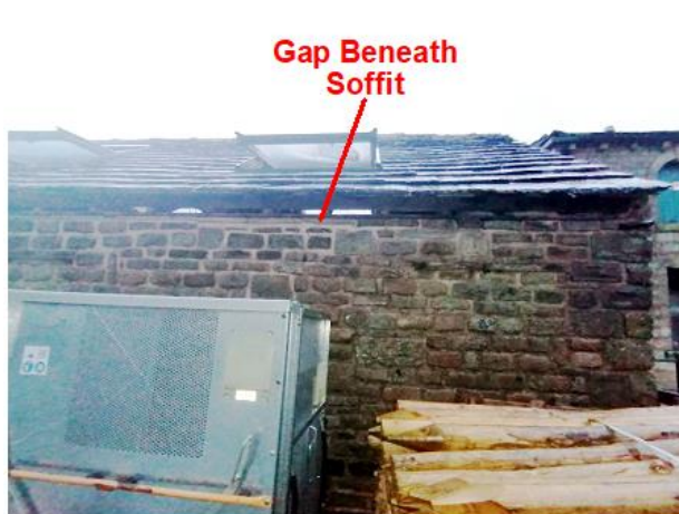
PHOTO 11 Western Henhouse Roof
