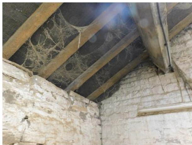
PHOTO 30 Underside of North-eastern Corner of Main Roof
