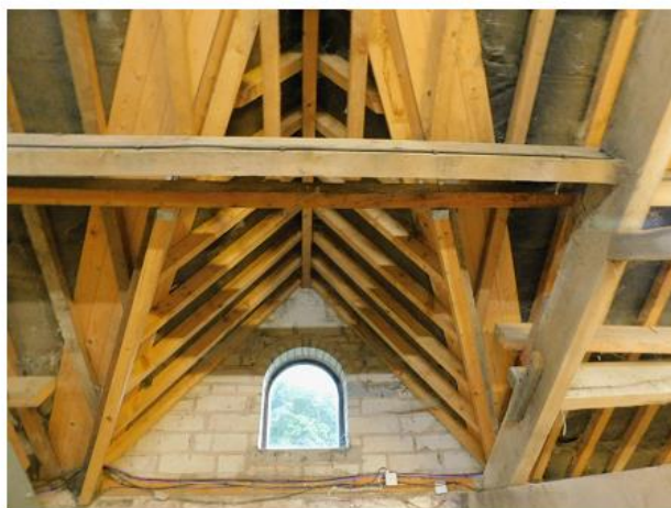
PHOTO 28 Underside of Southern Dormer Roof
