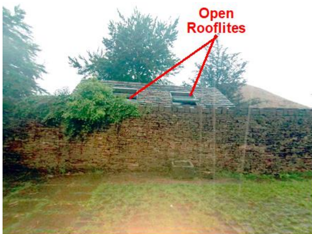
PHOTO 13 Eastern Elevation of Henhouse
