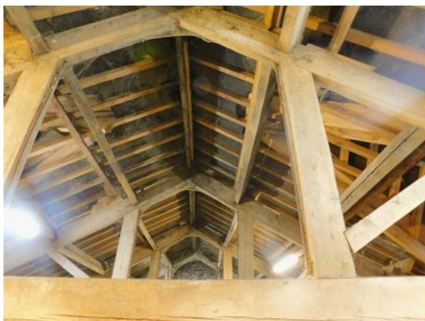
PHOTO 25 Underside of Central Roof
