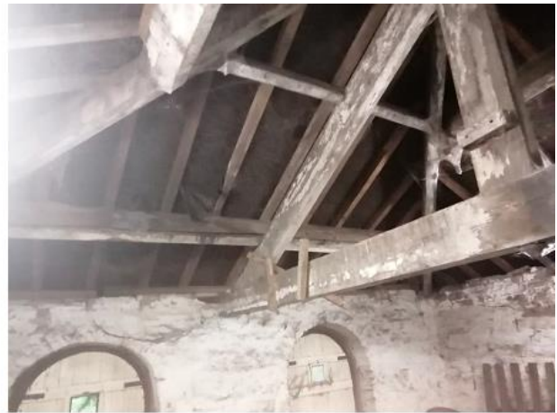
PHOTO 32 Underside of the Internal North-eastern Roof
