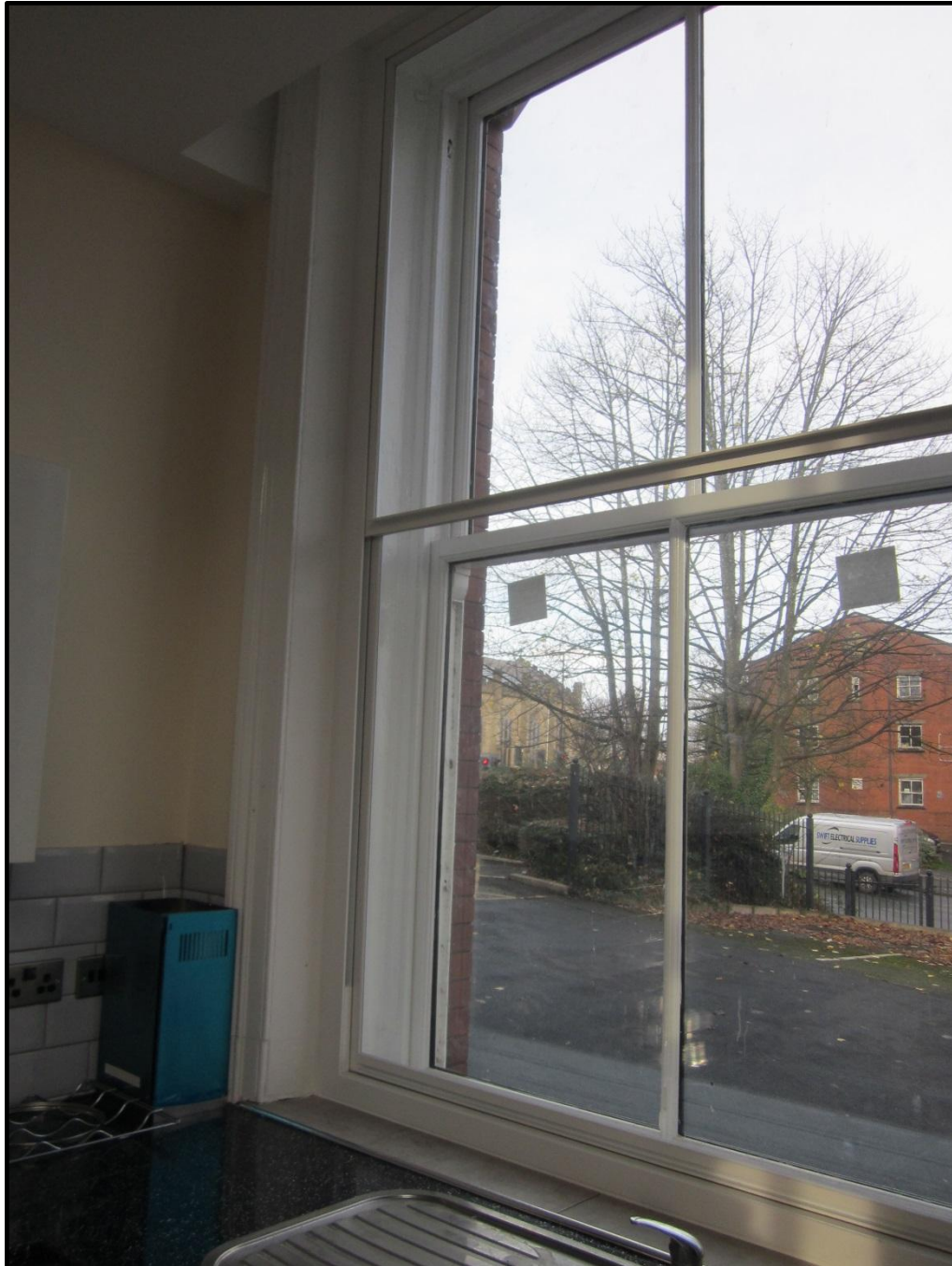
Photograph 7. Secondary glazing to the kitchen area of the living room/kitchen
