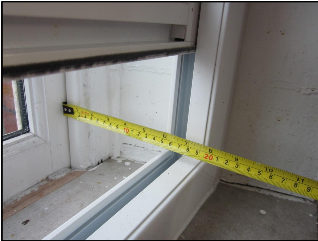
Photograph 8. Secondary glazing cavity, living room/kitchen
