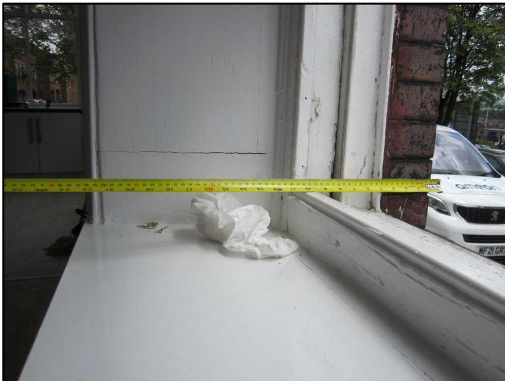
Photograph 6. External walls to the existing building
