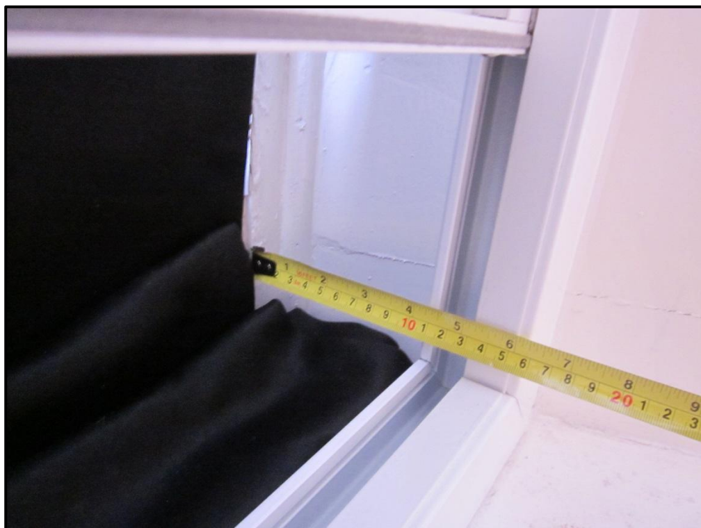
Photograph 10. Secondary glazing cavity, bedroom
