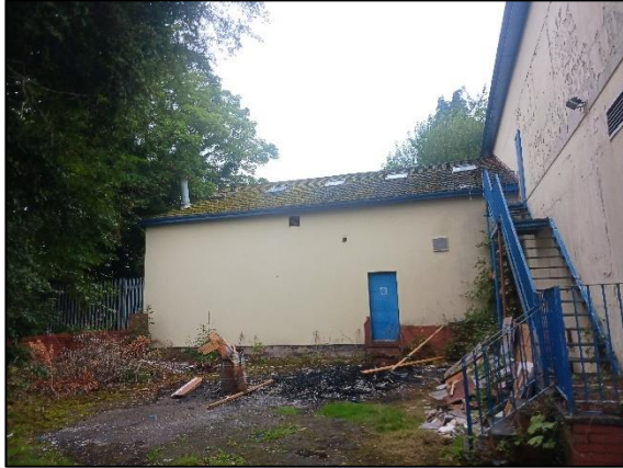
Figure 2.6: View of the south elevation of the single storey element and parking / hardstanding area.
