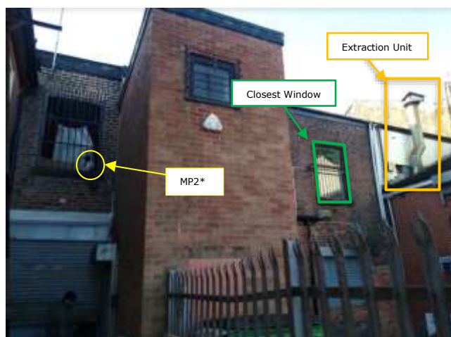
Figure 3.0 – Rear Façade and extraction unit from the commercial development.
