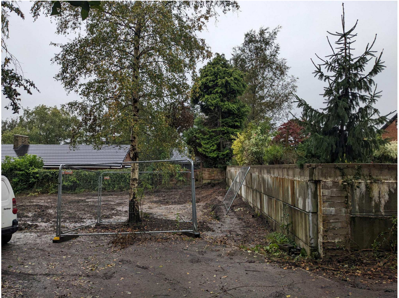
Photograph 2: The north-western part of the site where the excavation occurred. T1 is visible to the right of frame, enclosed by heras fencing.
