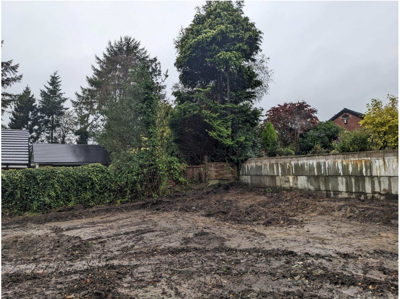
Photograph 3: A view of the area where the excavations were undertaken in the north-western part of the site.
