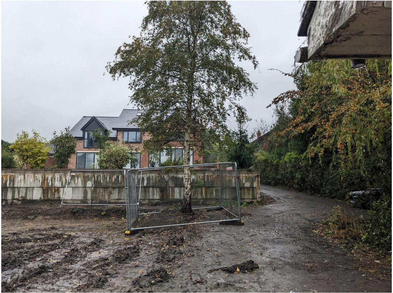
Photograph 1: The north-western part of the site where the excavation occurred. T1 is visible to the right of frame, enclosed by heras fencing.
