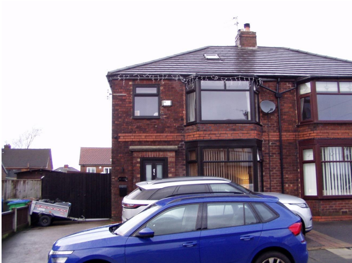
View of front of property from Glamis Avenue
