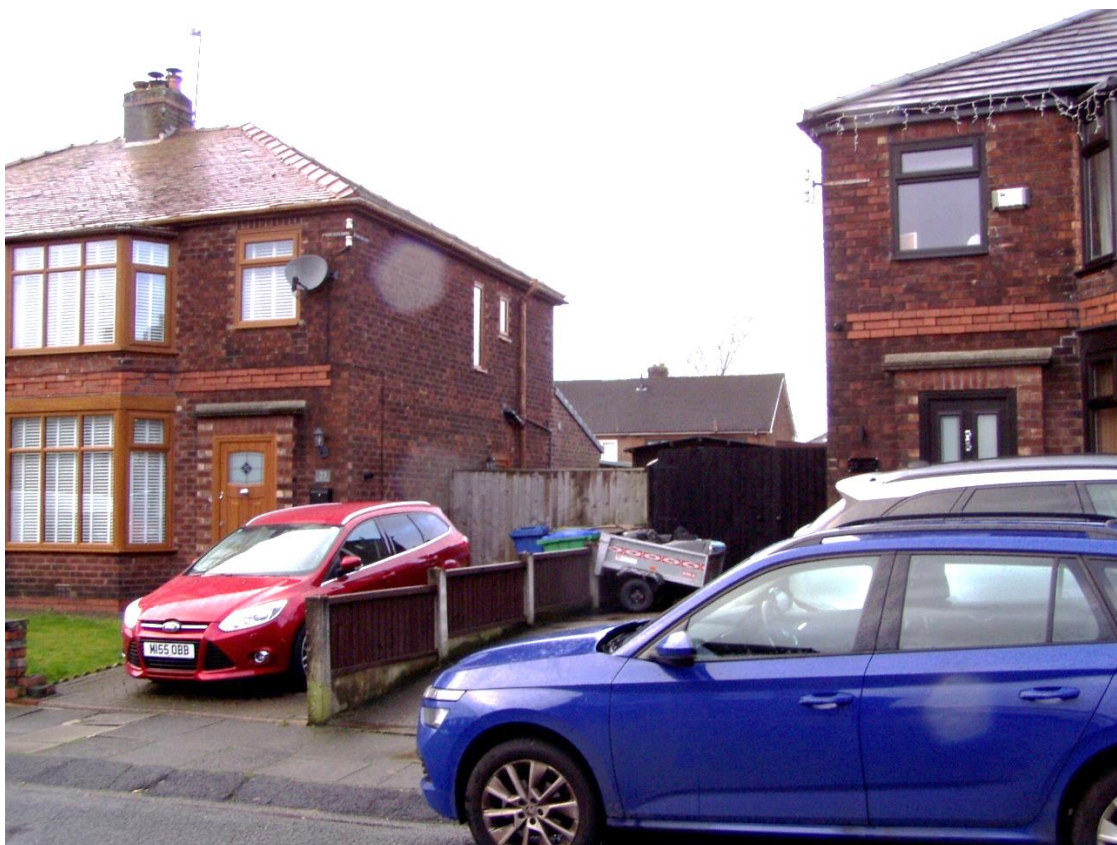
View of front of property from Glamis Avenue showing relationship between number 25 and number 23 to the left.
