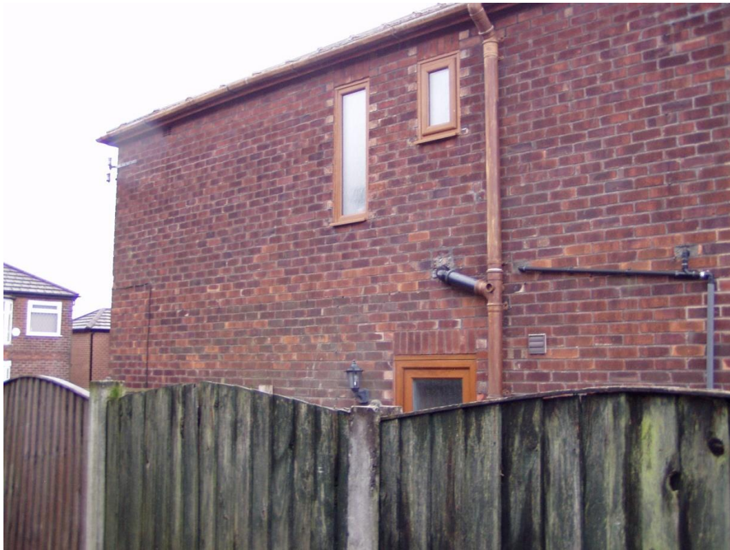
View of side elevation of number 23 Glamis Avenue from side garden of number 25.
