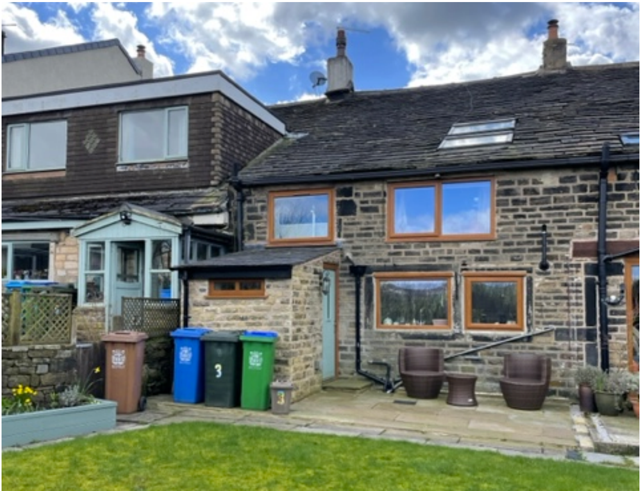
Existing rear elevation showing small porch sized extension that the client wants to remove for the proposed new single level extension
