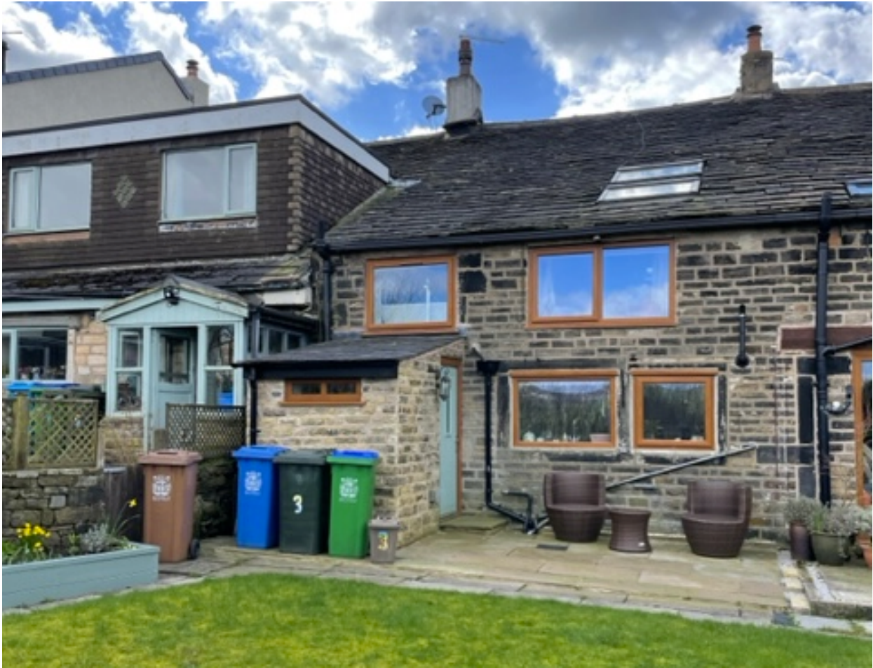
Existing rear elevation image of No 5 showing various extensions and alterations, with rear elevation of No 3 to the right
