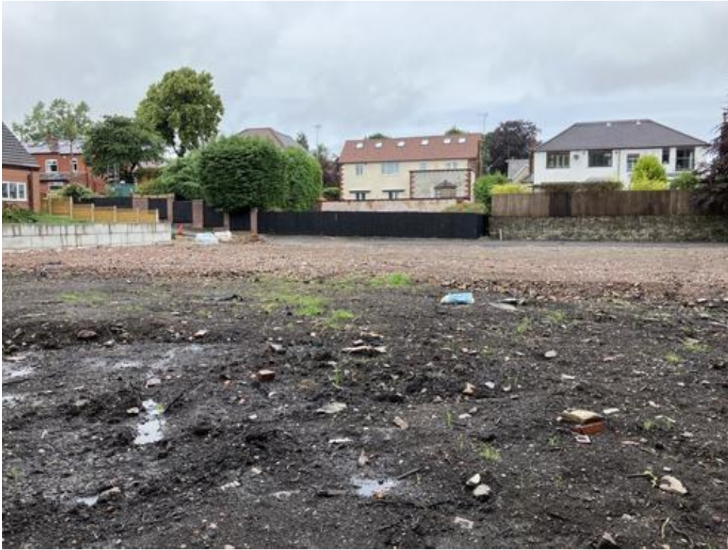
PLATE 3 VIEW OF SITE FACING NORTH
