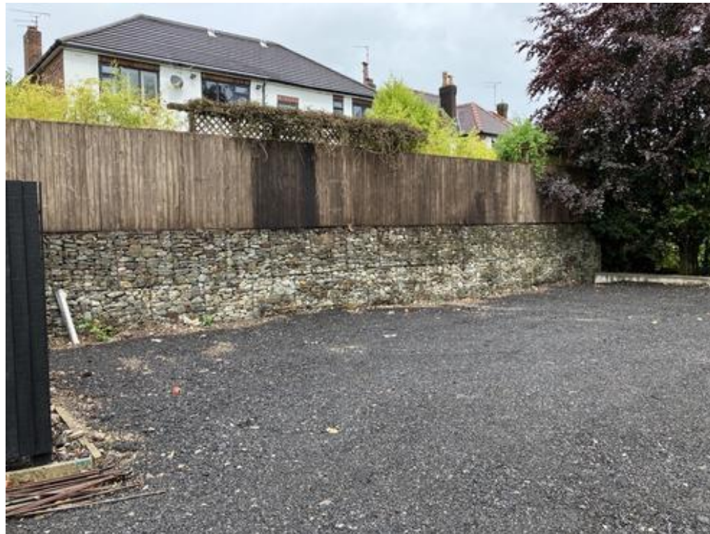
PLATE 4 GABION WALL – NORTHERN BOUNDARY
