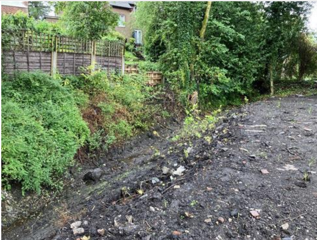
PLATE 2 EMBANKMENT TO STREAM ALONG THE SOUTHEAST BOUNDARY
