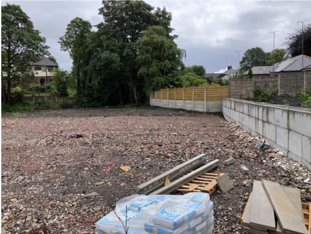
PLATE 5 CONCRETE RETAINING BLOCKS – WESTERN BOUNDARY
