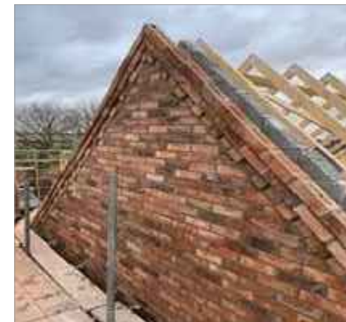
Verge brick corbel detail - Butterley carbon black smooth
