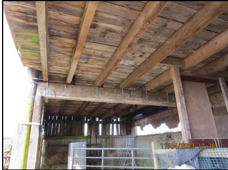
Photograph 091 Main stanchion and first floor support
