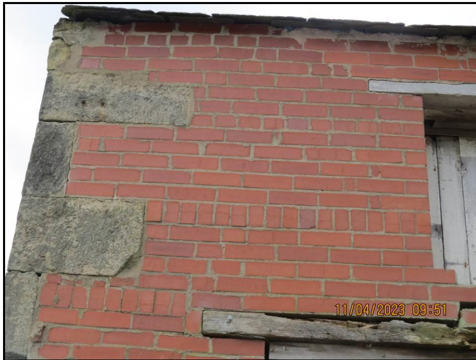
032 Satisfactory wall profile, chainage 0 – 2 metres
