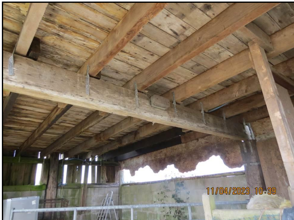
092 Cross beam support, rear wall
