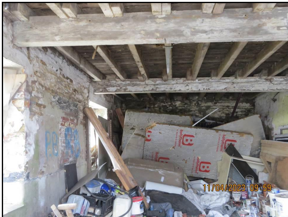
043 Ground floor, South East
