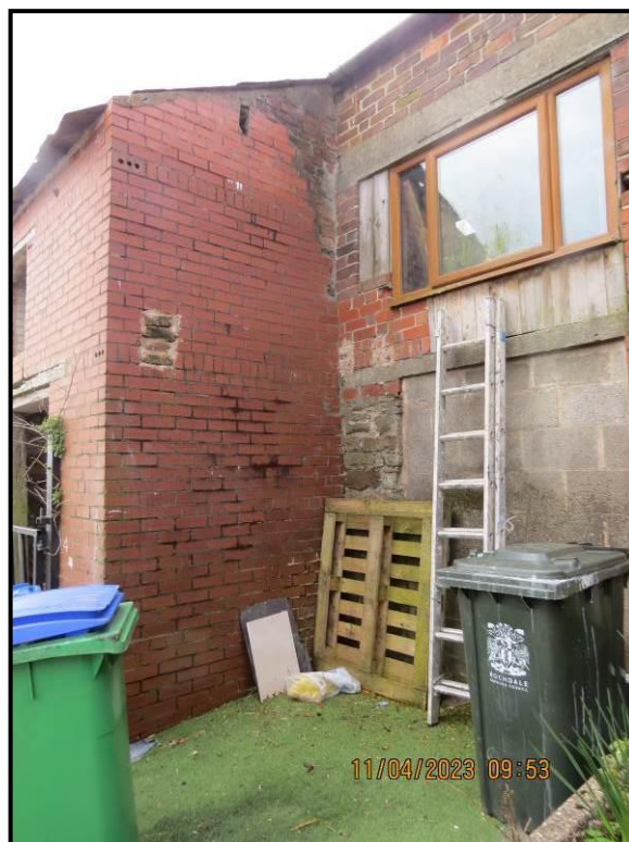
037 Return wall, chainage 4.5 metres
