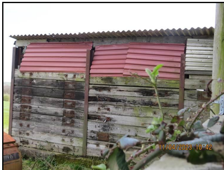
Photograph 096 External rear elevation (East)
