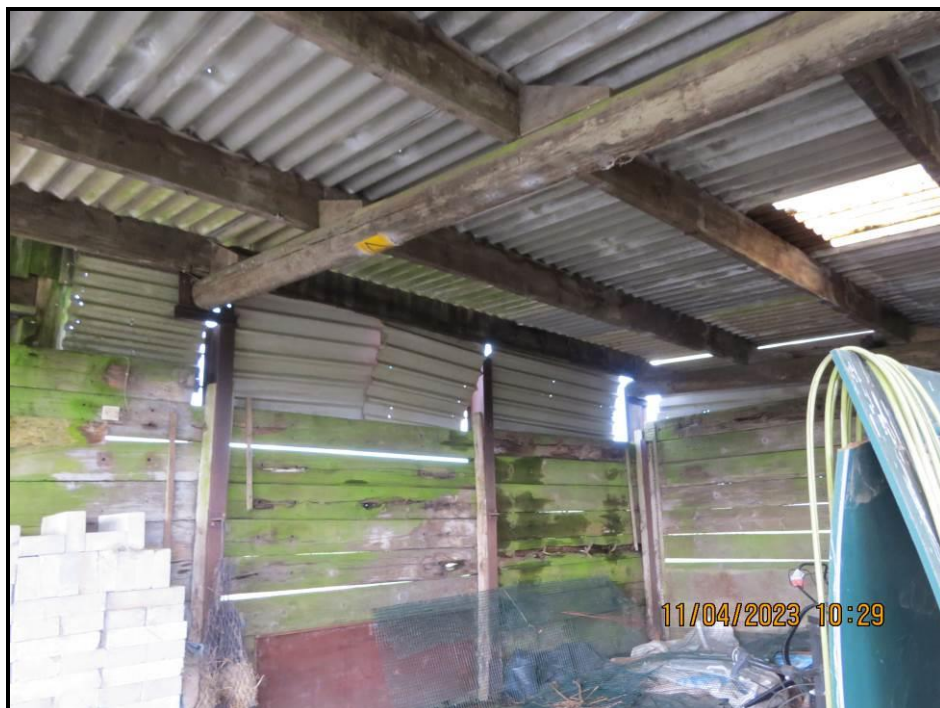
082 Ground floor gable to barn (East)
