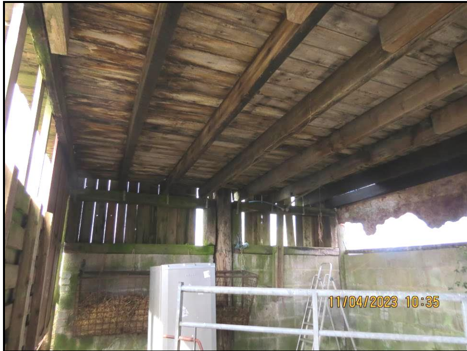
089 Shippon, ground floor looking South East – North West
