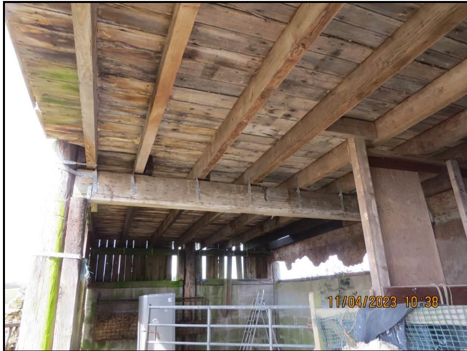
091 Main stanchion and first floor support
