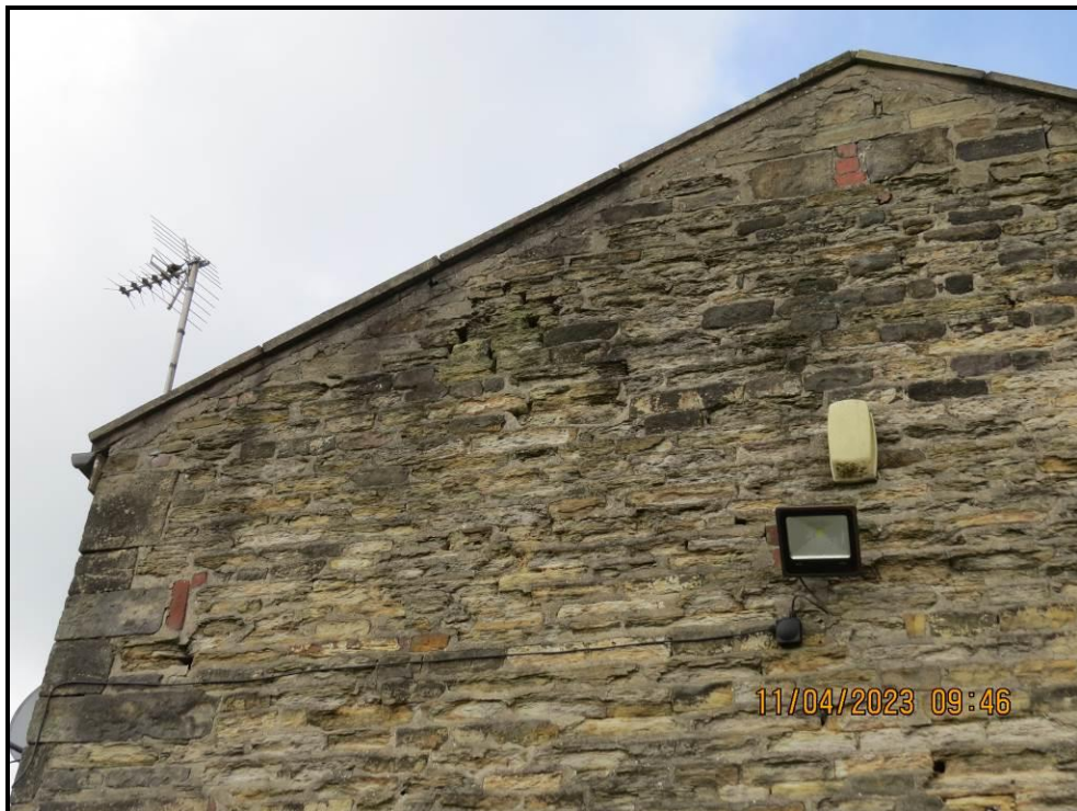
024 Upper gable, chainage 0 – 4 metres
