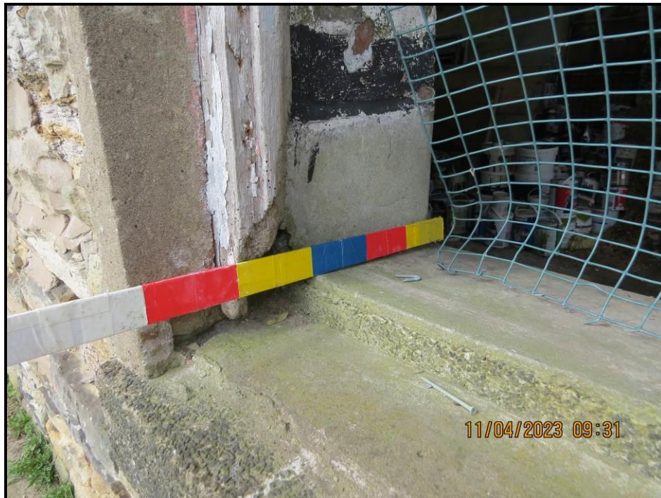
007 Gable wall depth
