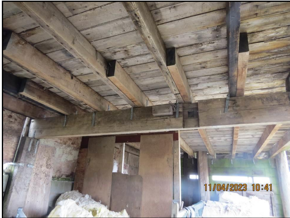
095 Floor beam and first floor looking North West – South East
