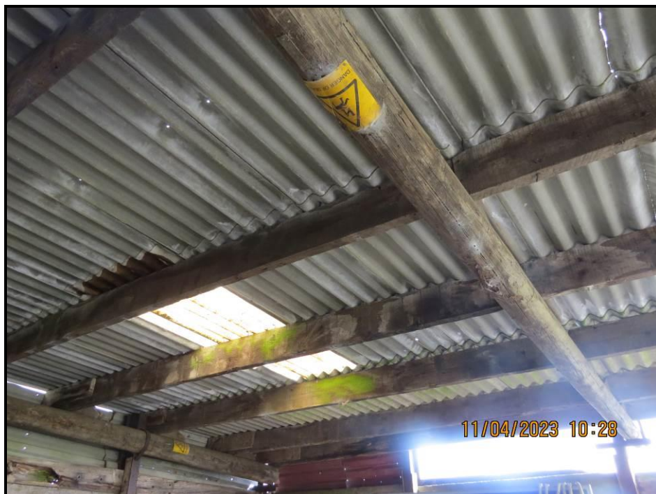
080 Main roof beam
