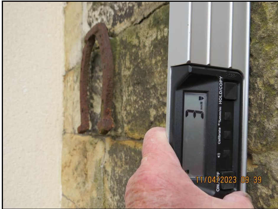
014 Good vertical alignment, chainage 1 metre
