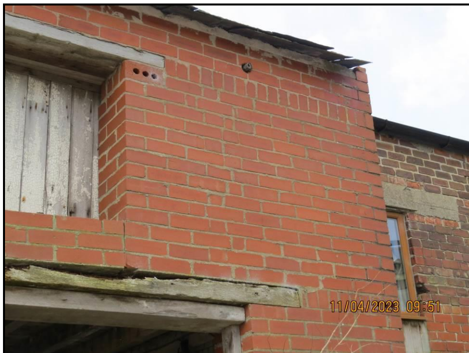
033 Satisfactory wall profile, chainage 3 – 4.3 metres
