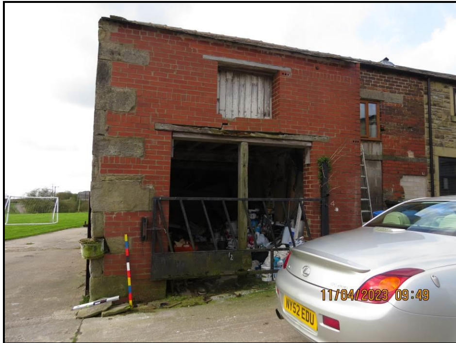
030 North West flank, chainage 0 – 4.3 metres
