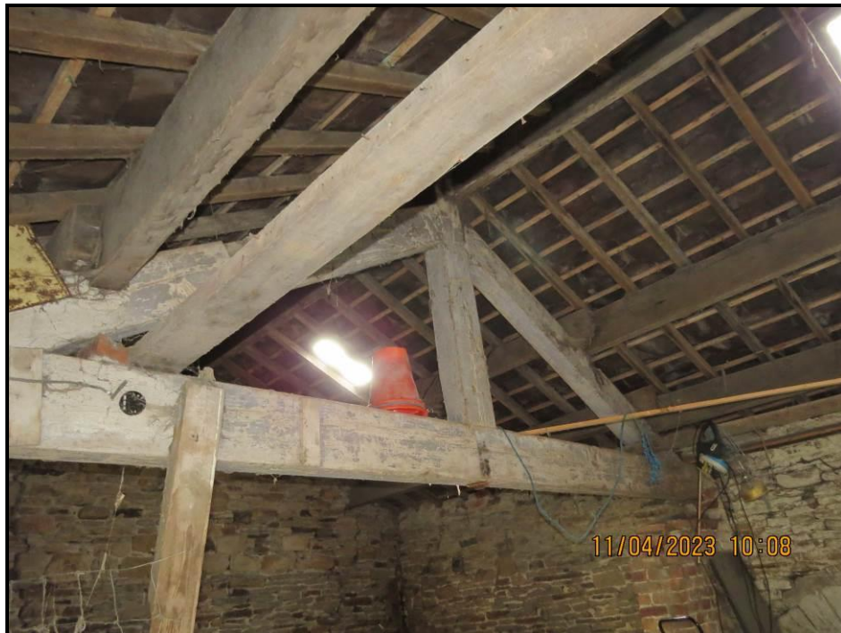
061 King post truss
