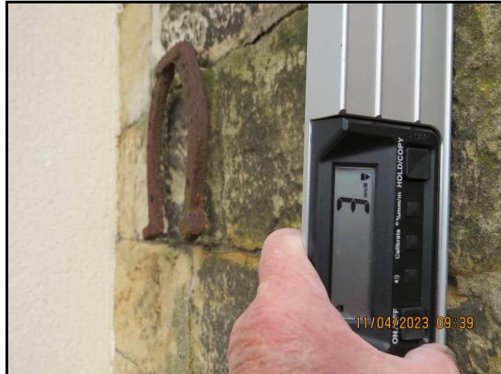
Photograph 014 Good vertical alignment, chainage 1 metre
