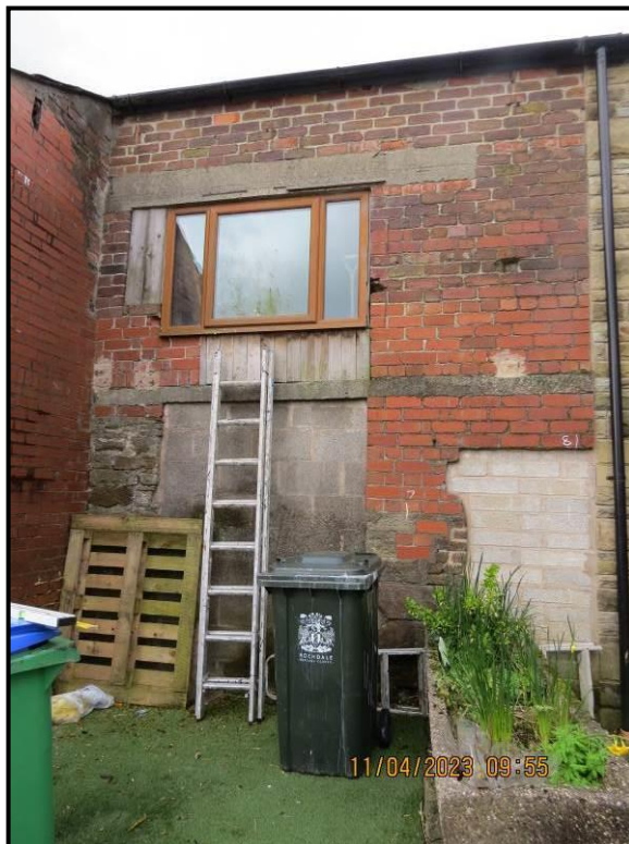
039 North East flank, chainage 5 – 8 metres
