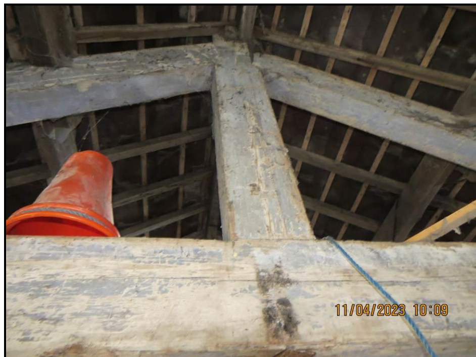
064 King post truss detail
