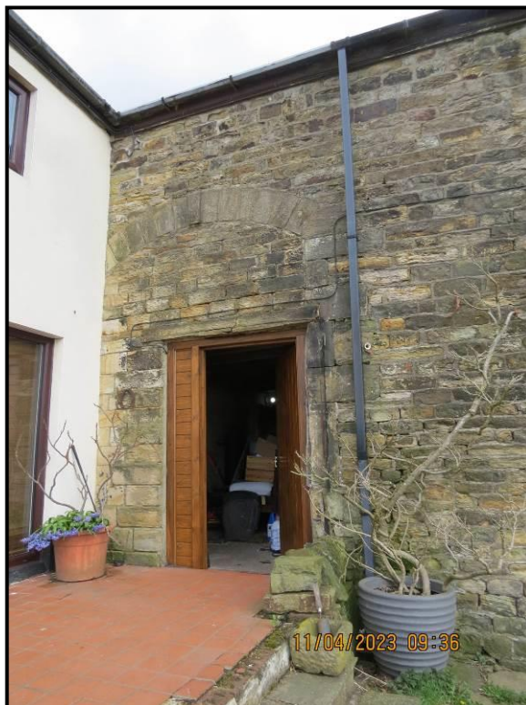
010 South West flank, chainage 0 – 3 metres
