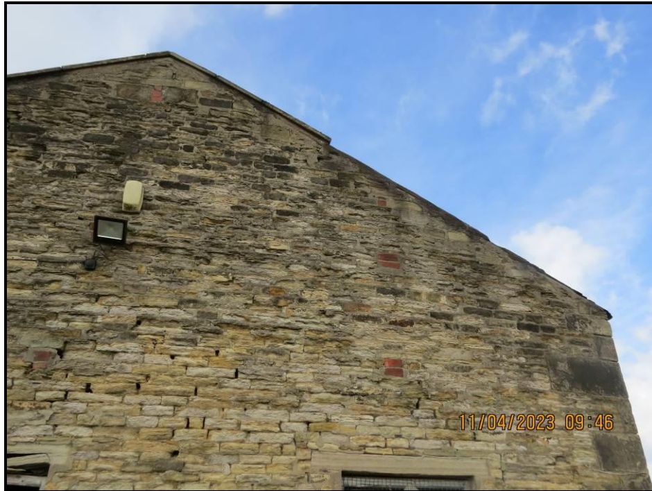
025 Upper gable, chainage 3 – 8 metres
