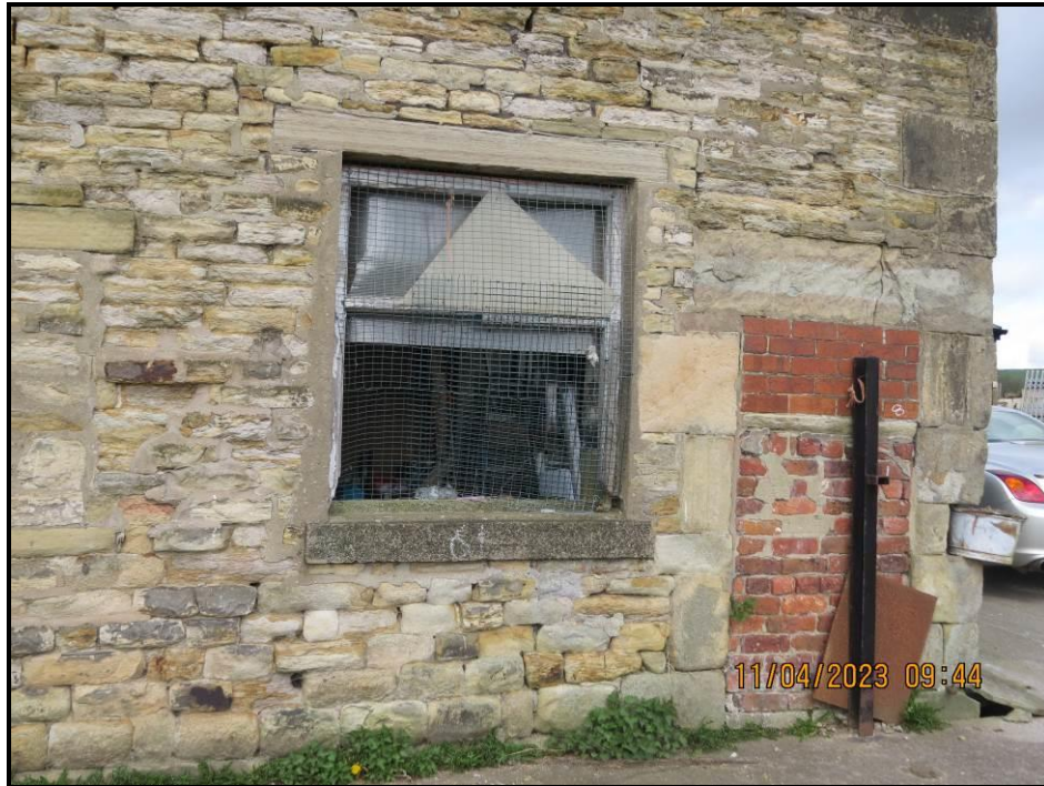
021 Gable, ground floor, chainage 5 – 8.20 metres
