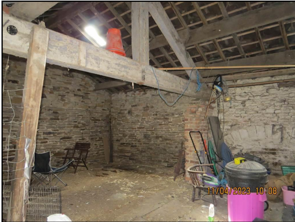
058 King post truss looking West – East
