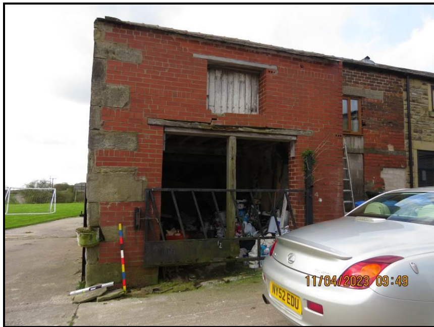
Photograph 030 North West flank, chainage 0 – 43 metres
