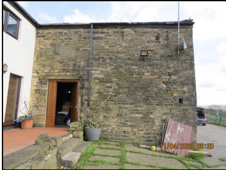
Photograph 006 South West flank wall
