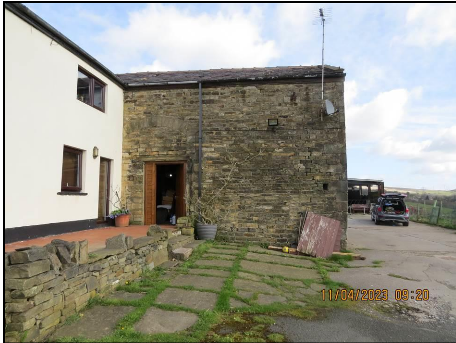
005 South West flank wall
