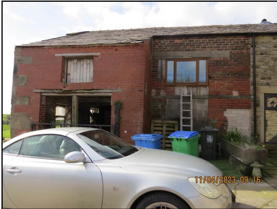
003 North East flank wall
