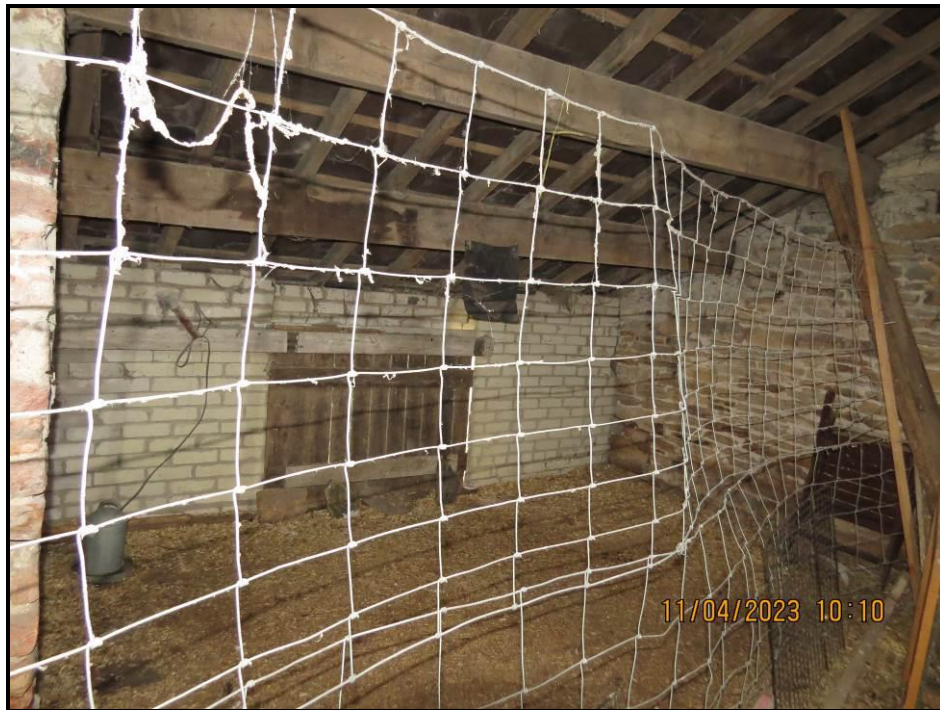
065 North East flank wall and South East gable
