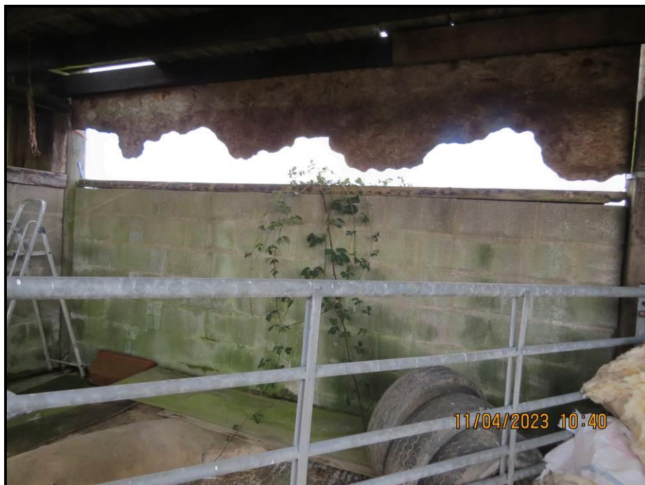
094 Blockwork plinth wall, rear elevation
