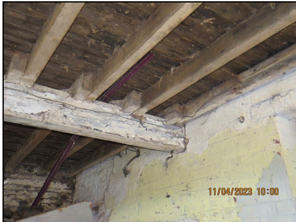
048 Satisfactory beam seating
