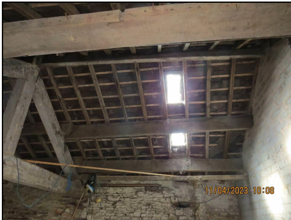
060 South West roof slope
