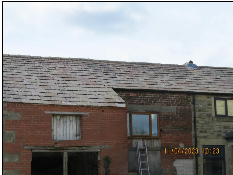
073 Satisfactory roof profile
