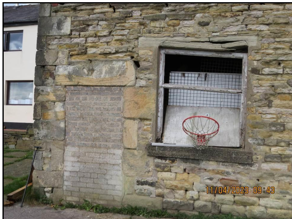
020 Gable, ground floor, chainage 0 – 3.5 metres
