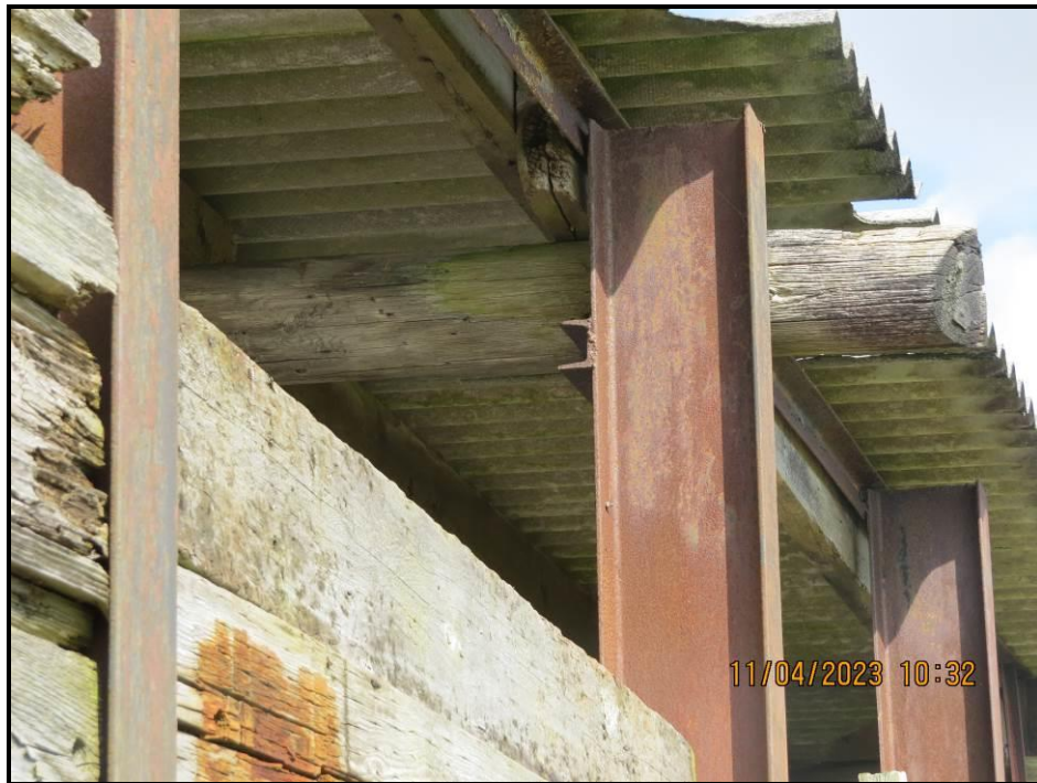
087 Typical stanchion deformation
