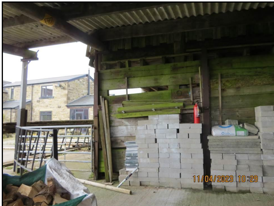
084 Ground floor gable to barn, chainage 0 – 3 metres
