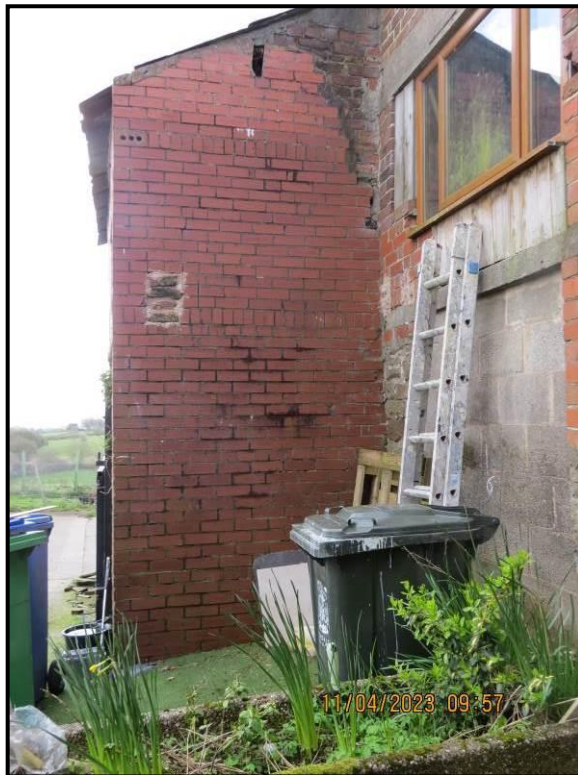
042 North West rear wall, chainage 0 – 2 metres
