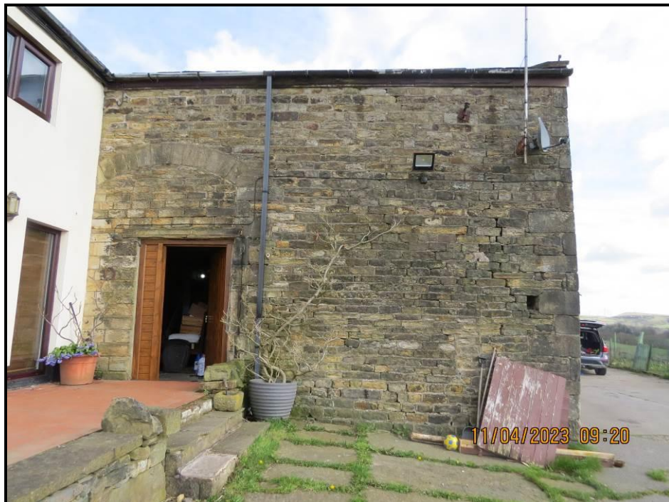
006 South West flank wall
