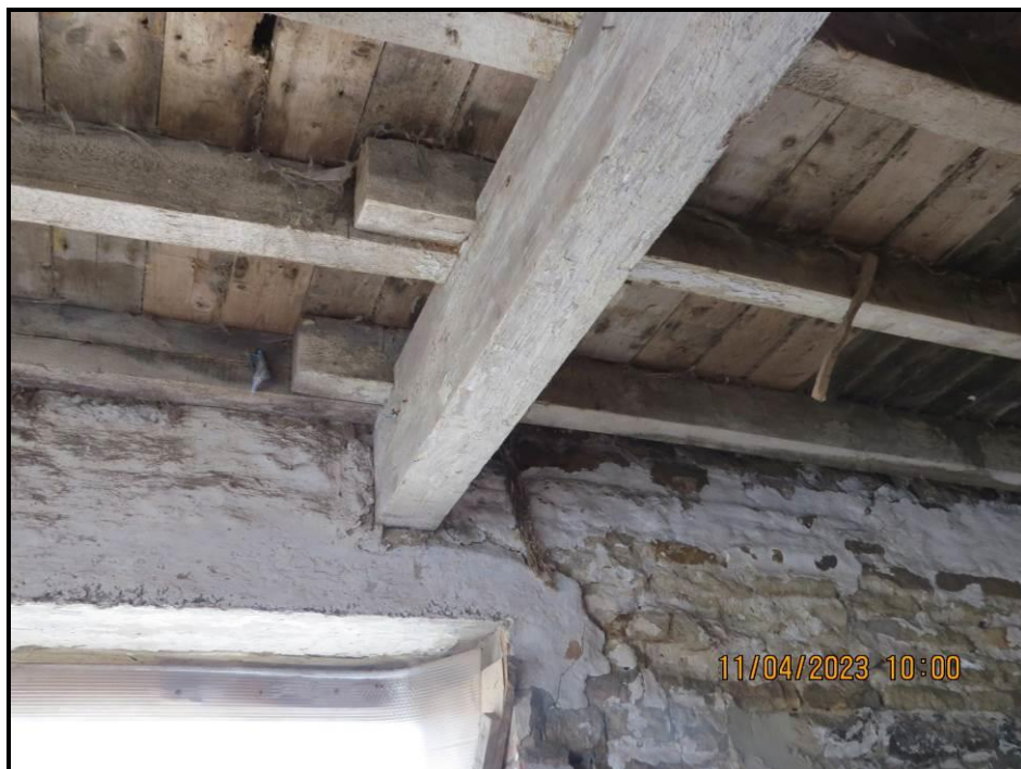
047 Satisfactory beam seating
