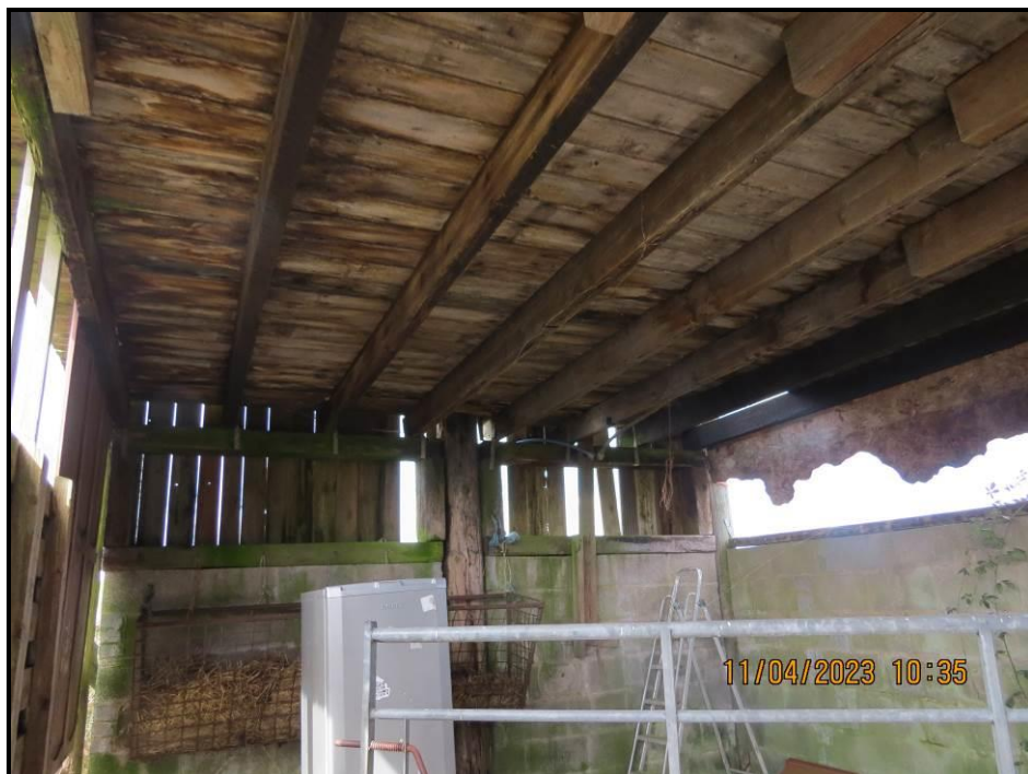
088 Shippon, ground floor looking South East – North West
