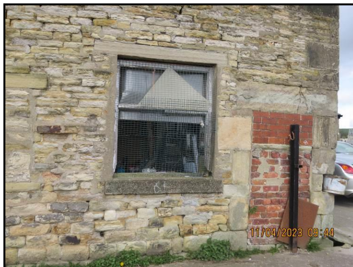
Photograph 021 Gable, ground floor, chainage 5 – 8.20 metres
