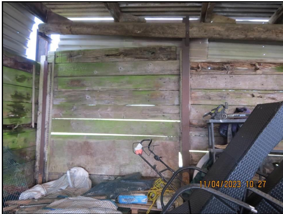
079 Rear wall (North West)
