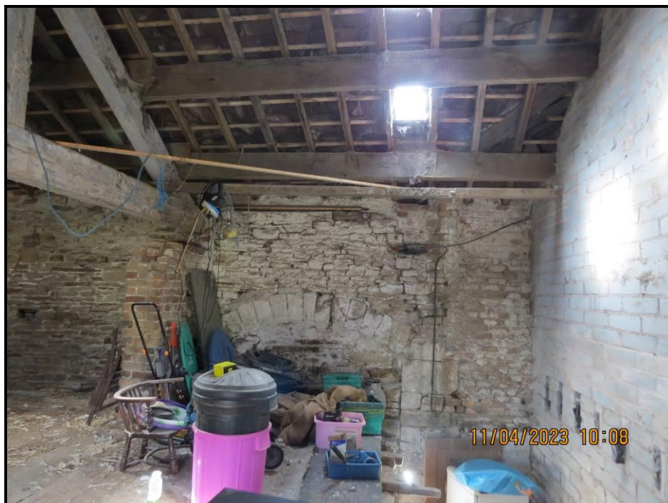
057 First floor, South West flank wall
