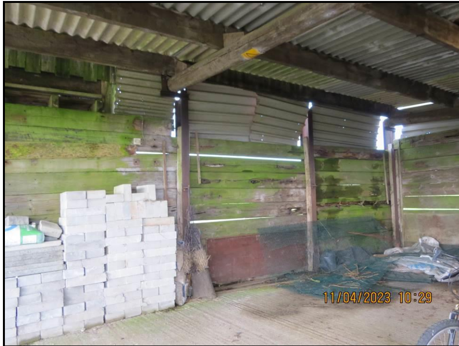
083 Ground floor gable to barn (West)
