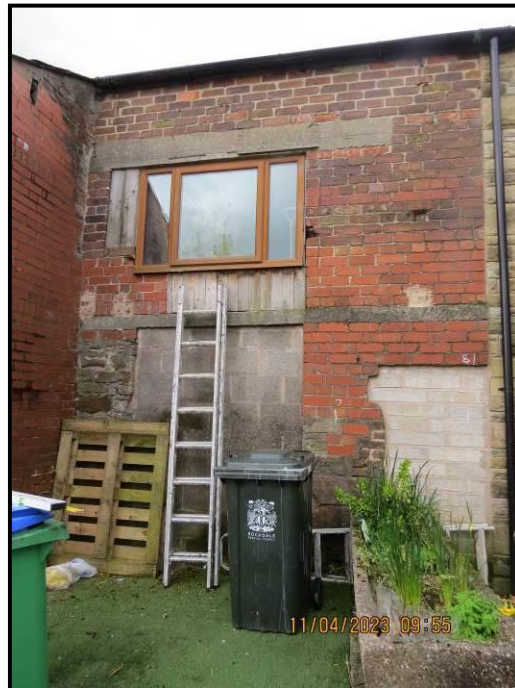
Photograph 039 North East flank, chainage 5 – 8 metres
