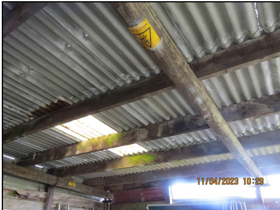
081 Main roof beam
