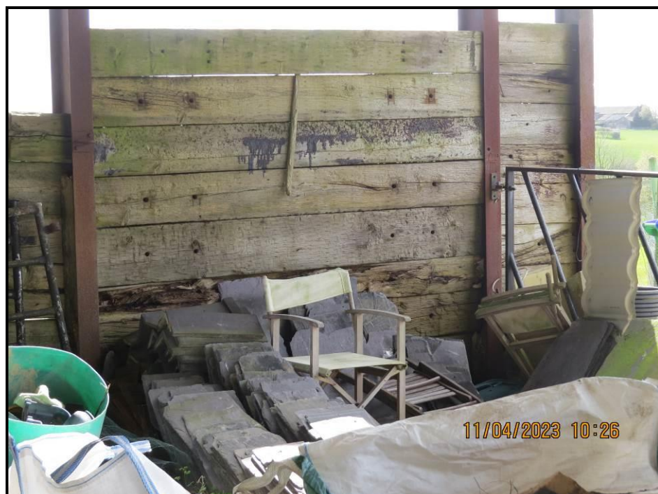
074 North East flank, stanchion – whaling detail
