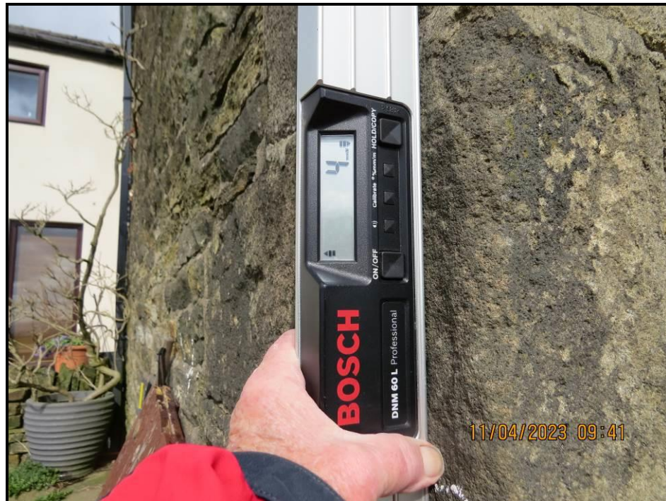
018 Good vertical alignment, South West corner
