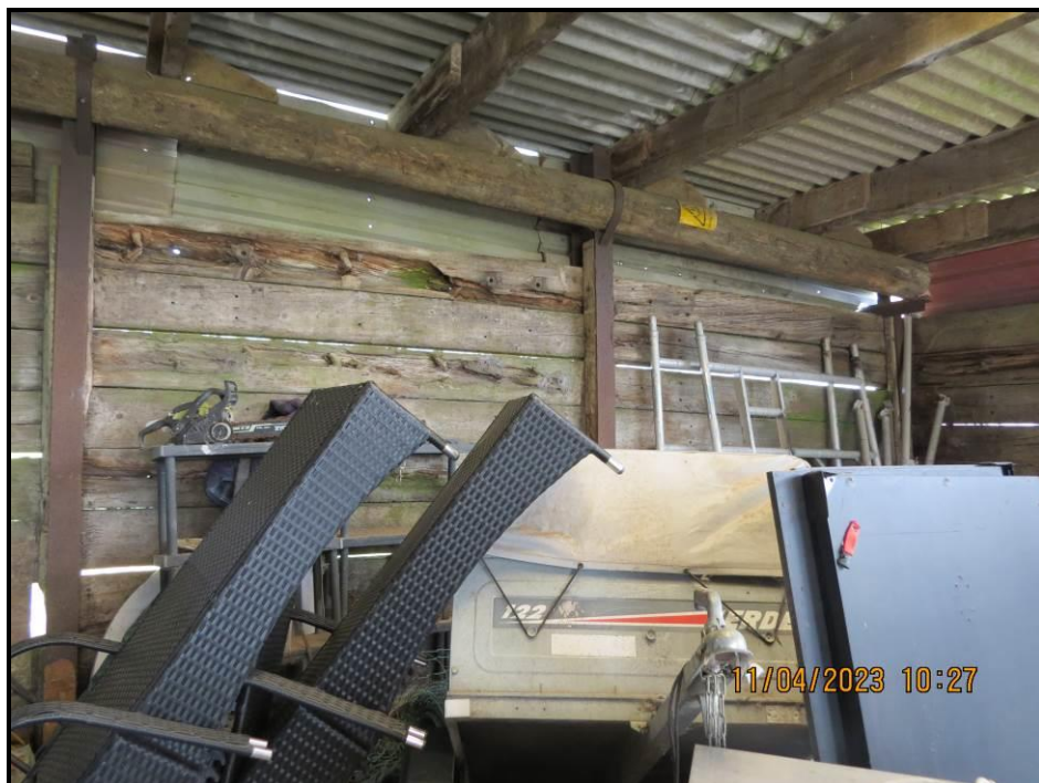
078 Rear wall (North West)
