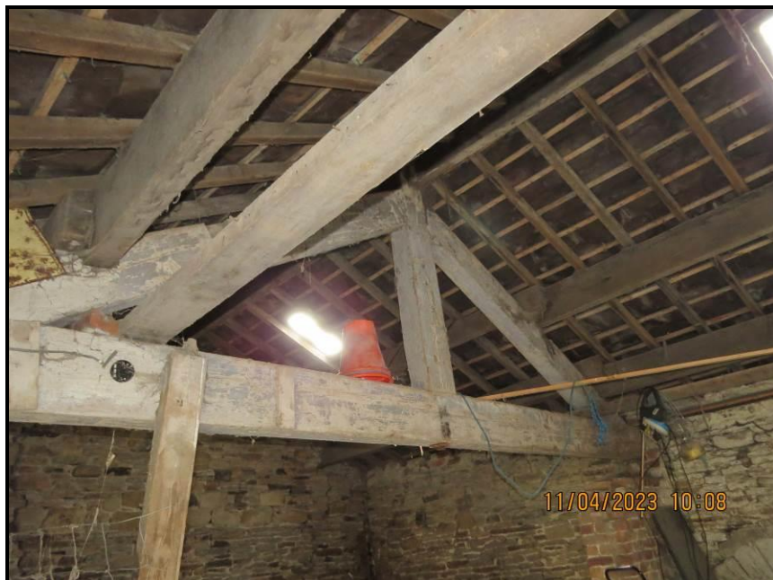
Photograph 061 King post truss
