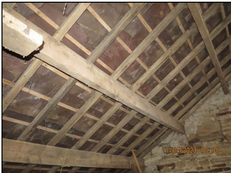
066 Purlin/rafter detail (North East)
