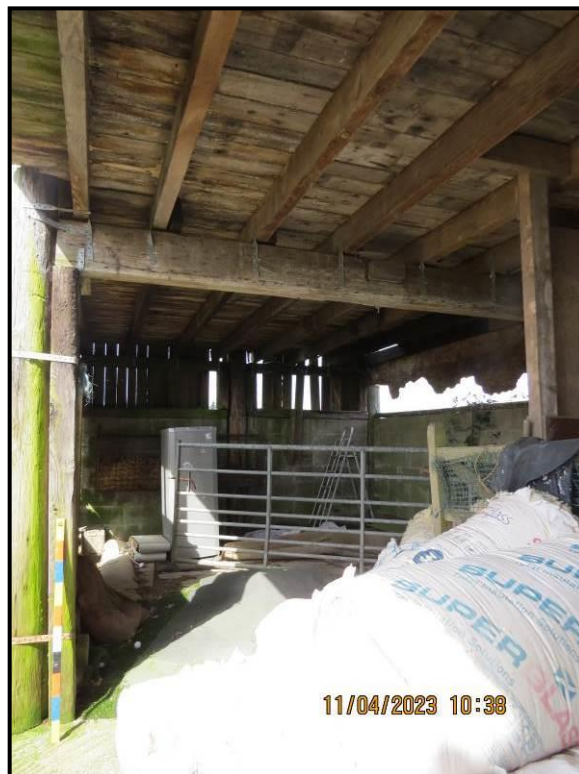
090 First floor support cross beam
