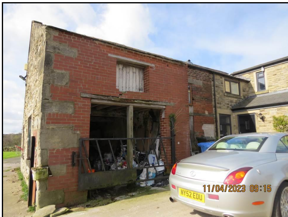
002 North East flank wall
