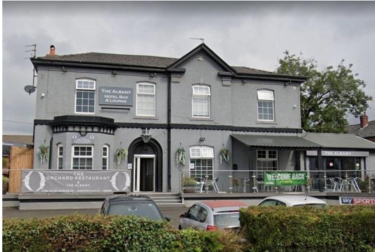
The Albany Hotel 87 – 89 Rochdale Road East Heywood Rochdale
