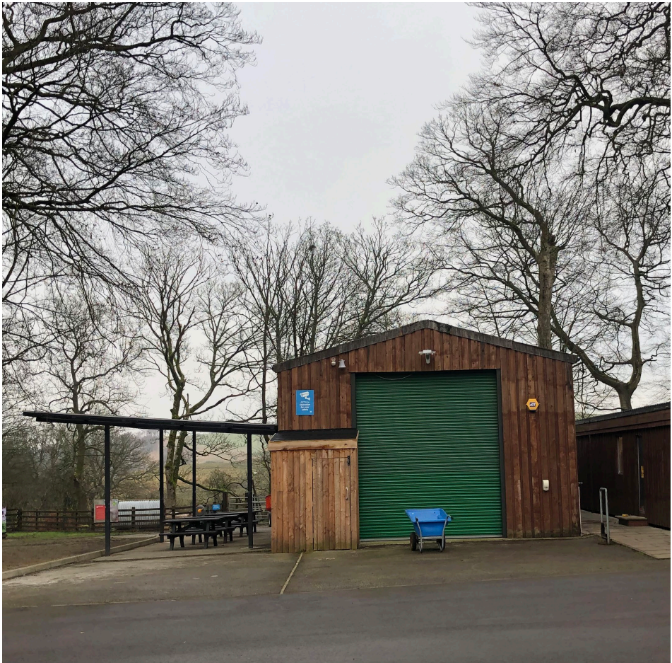
Item 1 - canopy and porch to shed
