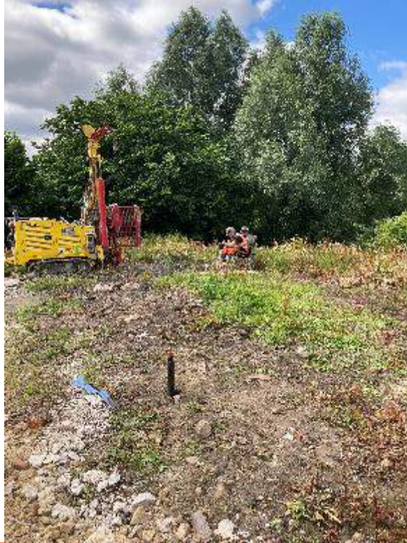
PLATE 7 MONITORING WELL INSTALL
