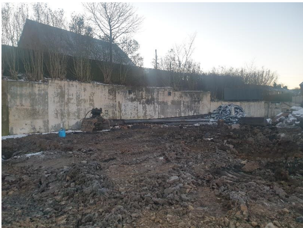
Photograph 2: Footprint of former building following demolition.
