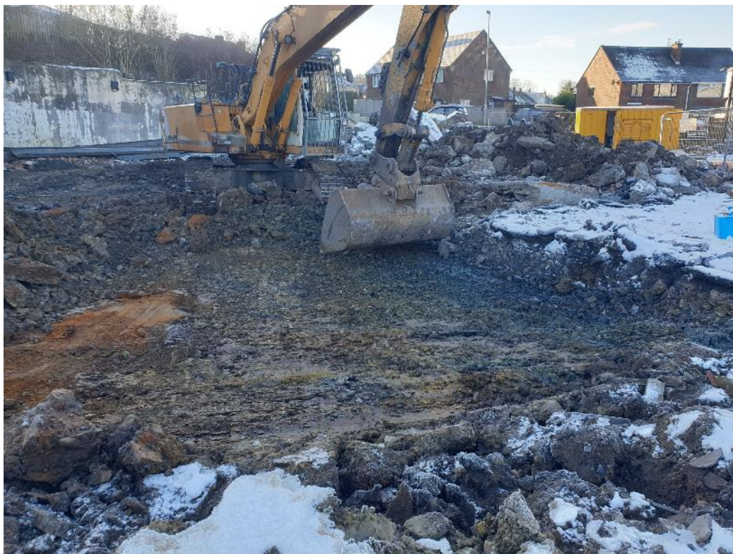
Photograph 4: Footprint of former building following demolition.
