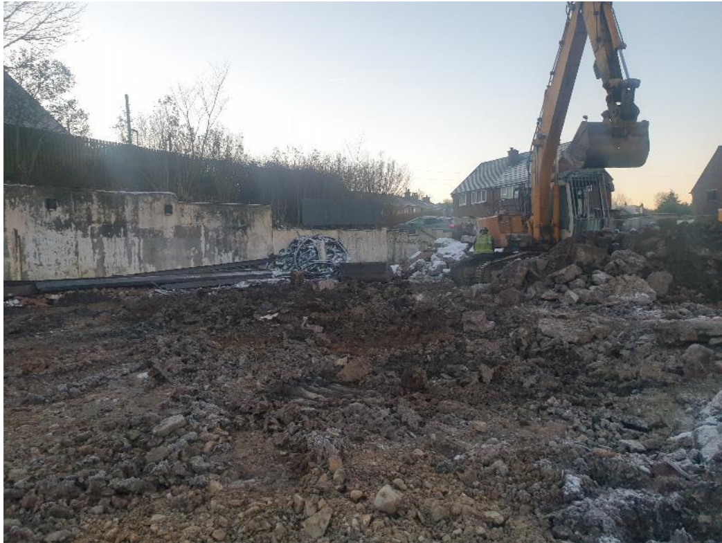
Photograph 1: Footprint of former building following demolition.
