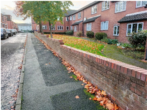
Left and Right – deteriorating wall on Fitton Street
