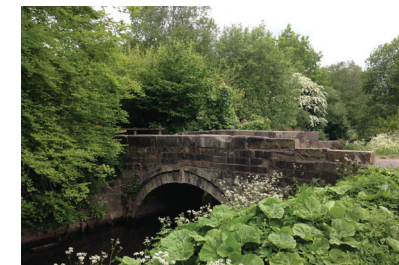
5. Grade II - Lever Bridge
