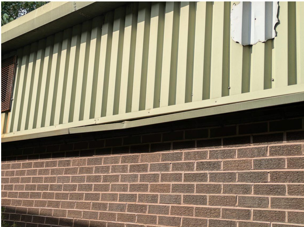
Plate 2: Image showing the damaged cladding on B3 .
