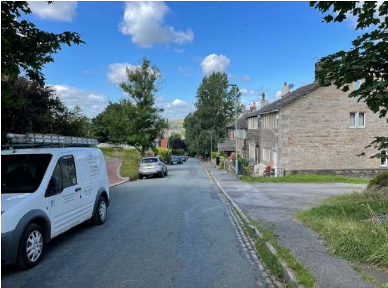
Figure 4.3: View of Blackstone Edge Old Road (August 2022)
