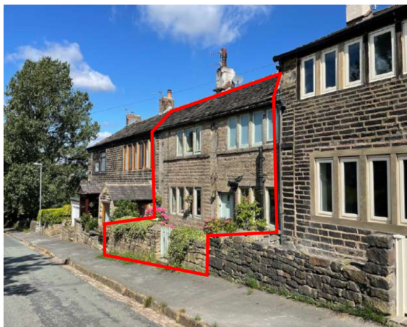
Figure 4.1: No. 5 Blackstone Edge Old Road (August 2022)
