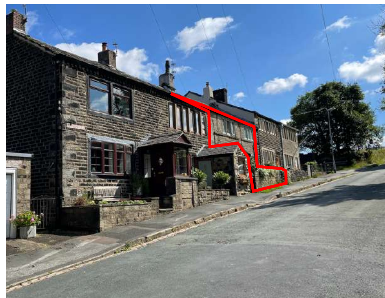
Figure 4.2: No. 5 Blackstone Edge Old Road (August 2022)
