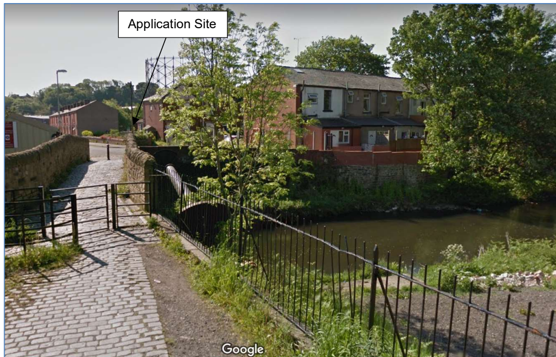
Figure 2. River Roch at Corporation Road, Rochdale (view south-east, extracted from Google Streetview)
