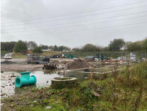
Photograph 1 – Proposed site compound.
