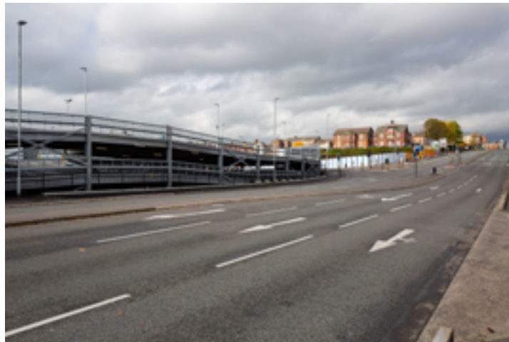
Figure 22 View D Pre-Construction of Rochdale Riverside Phase 2 (2020)
