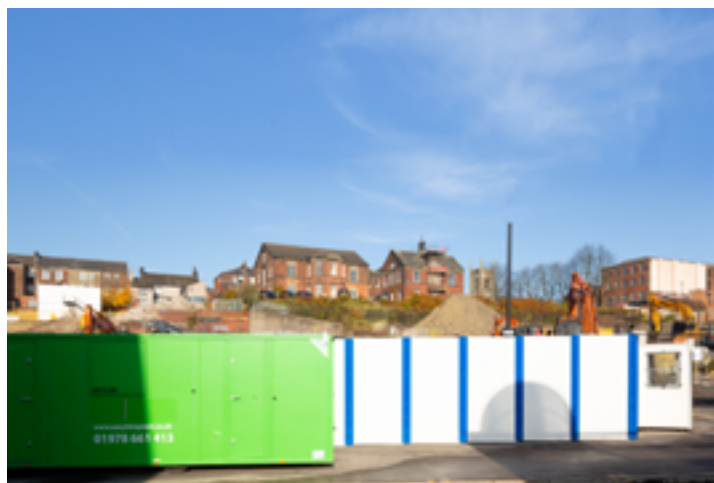
Figure 20 View F Pre-Construction of Rochdale Riverside Phase 2 (2020)
