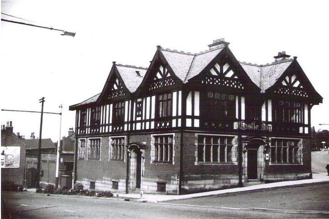
Figure 2. Historic Image of the Replacement Castle Inn Circa 1970 (Source: Judith Lucas)
