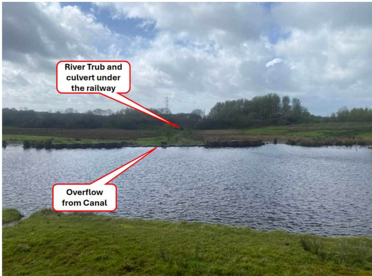
Figure 2: Picture of the Overflow Channel
