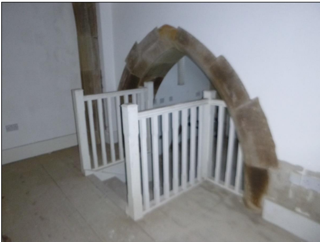
Fig.14 - Retained stone details to House 1
