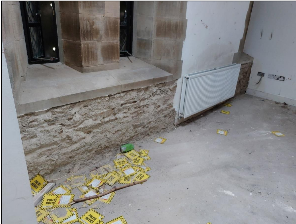
Fig.19 – Missing plaster
