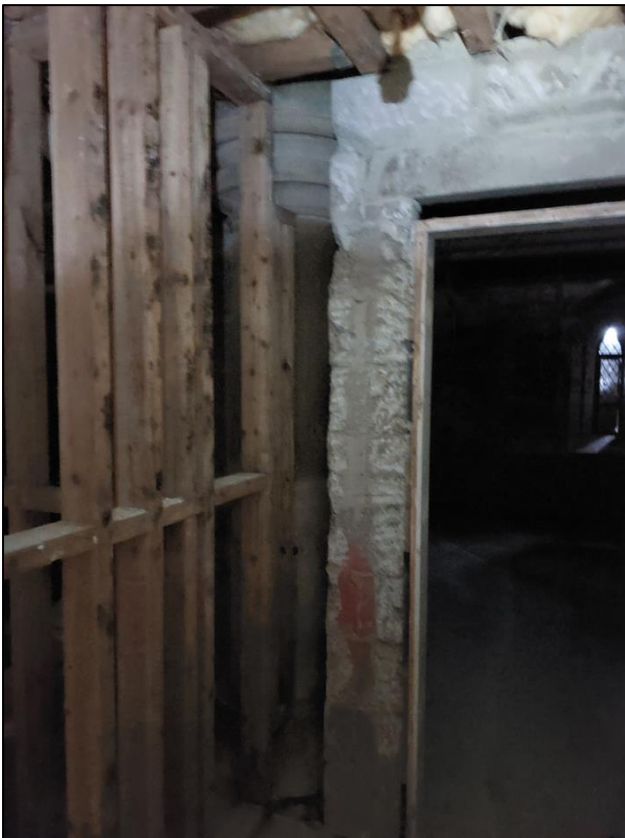
Fig.8 – Stone column No. 8 in House 2
