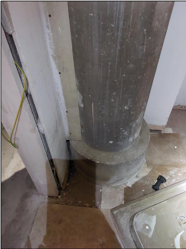
Fig.5 – Stone column No. 7 in House 4
