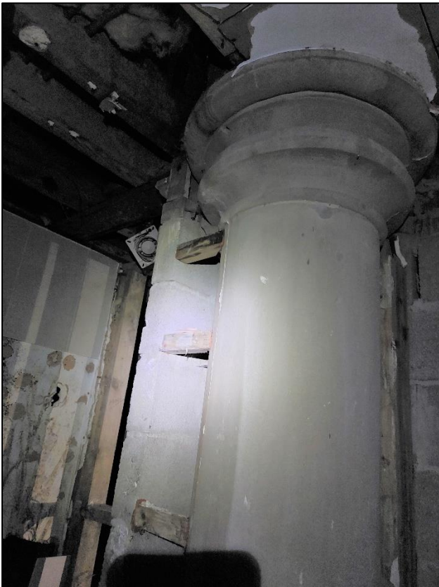
Fig.10 – Stone column No.5 in House 5
