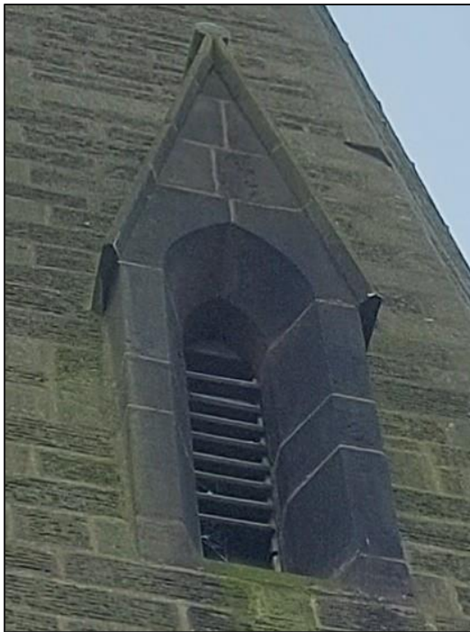
Fig.13 - North facing window, indicating timber louvres slots fixed within reveals.
