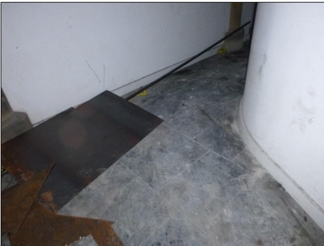
Fig.22 – Vinyl tiles within Entrance Hall
