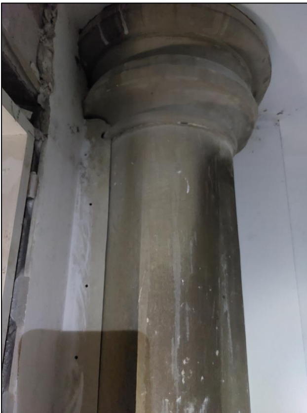
Fig.6 – Stone column No. 7 in House 4
