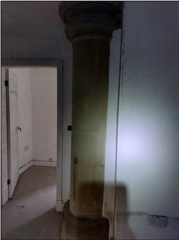
Fig.3 – Stone column No. 4 in House No.2
