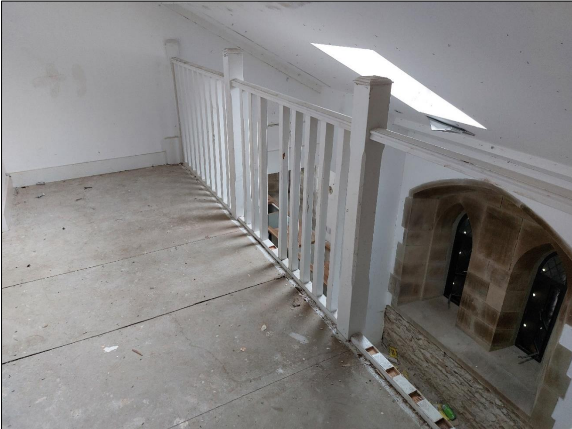
Fig.24 – Example of existing Balustrade
