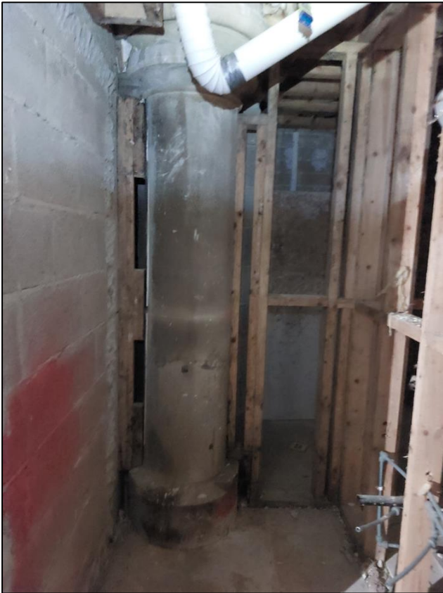
Fig.7 – Stone column No. 8 in House 2
