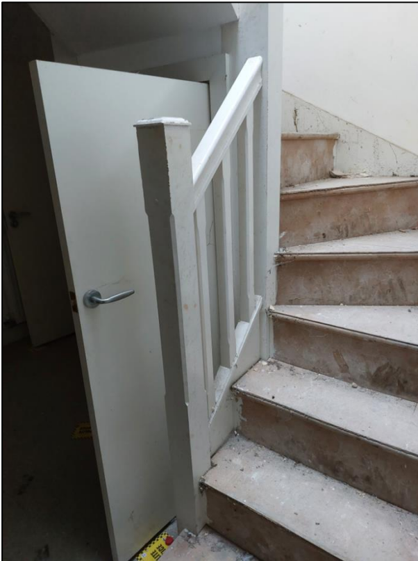
Fig.23 - Example of existing Balustrade
