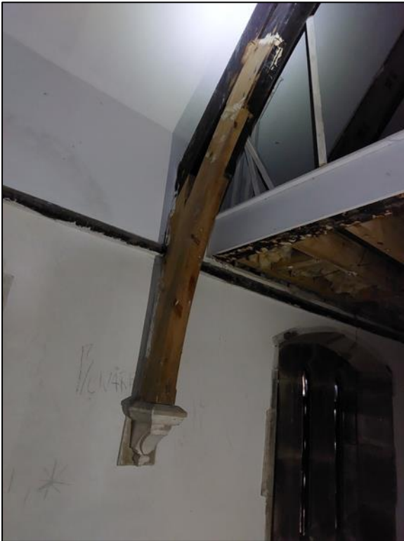
Fig.15 – Retained corbel with truss in House 2
