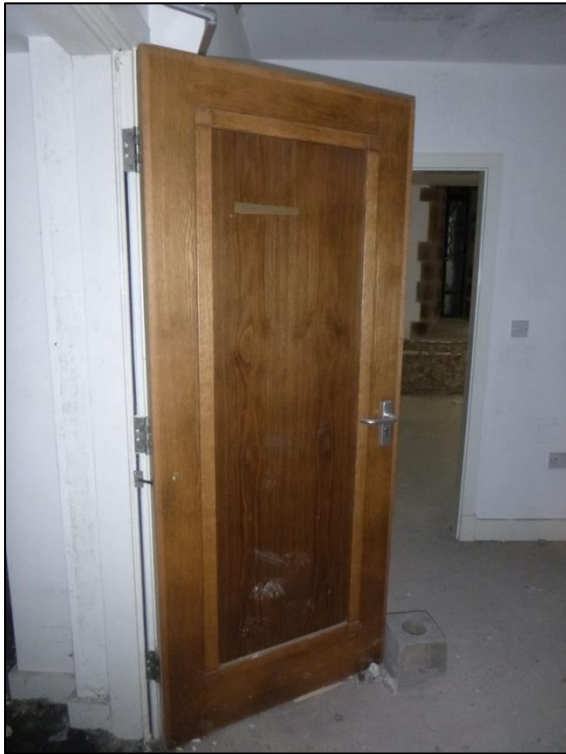
Fig.25 - Existing entrance door off Entrance Hall
