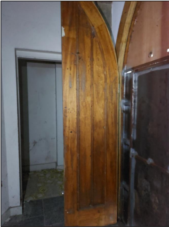
Fig.27 – Existing Nave door
