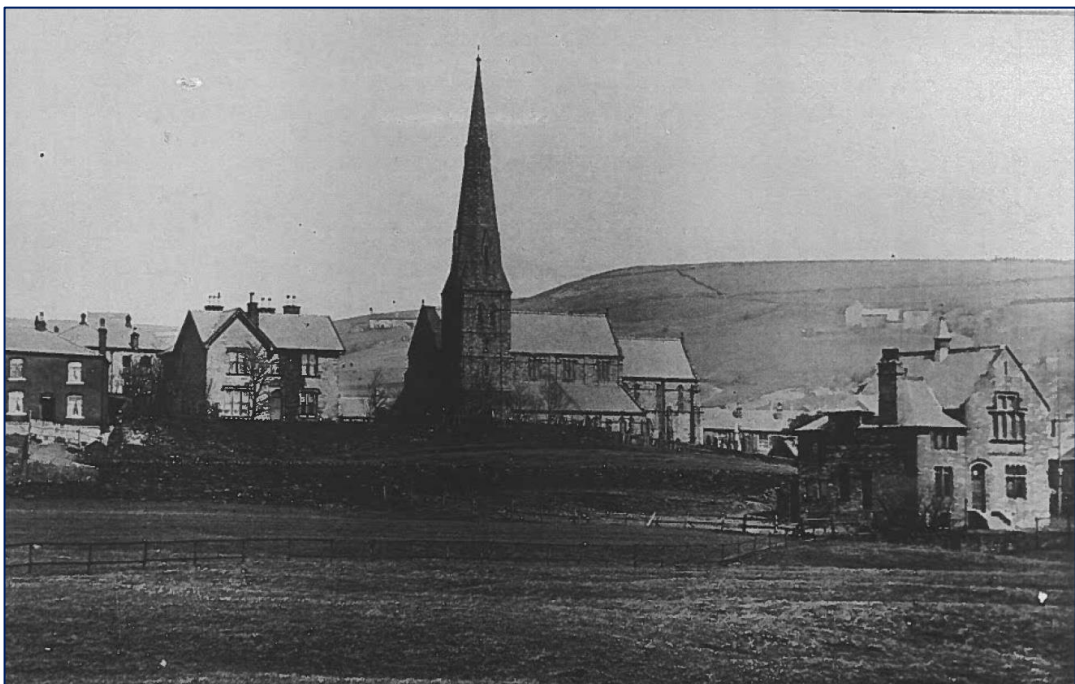
Fig.8 - Image from unknown date (Source: Your Trust Rochdale). South elevation of St James Church before the cemetery was expanded to the south elevation and the late 20 th century housing development was constructed. The detached building on the right-hand side of the picture was formerly called St James Tavern and appears to be a similar age to the church.
