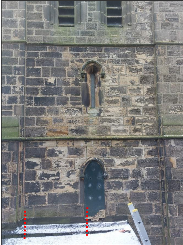
Fig.19 - Red lines indicate approximate width of door opening in context of the total width of the tower
