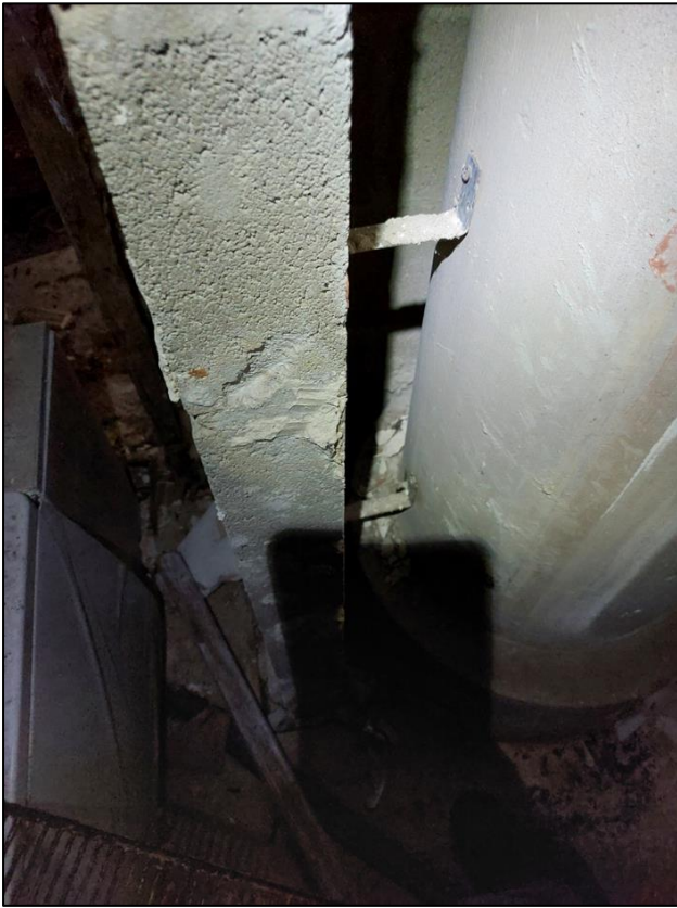
Fig.9 – Stone column No.5 in House 5
