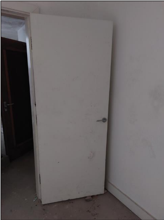
Fig.21 – Existing internal flush doors
