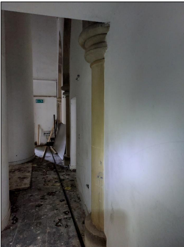
Fig.2 – Retained outline of stone columns 1-3 and stone arches within Entrance Hall
