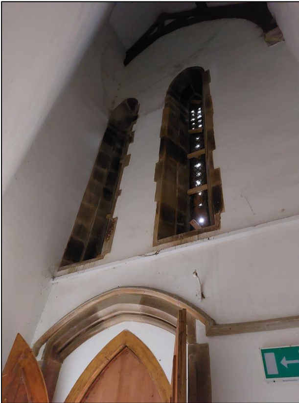
Fig.1 – Internal West elevation wall within Entrance Hall
