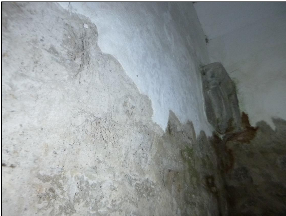
Fig.20 – Remnants of original 3-coat lime plaster to walls
