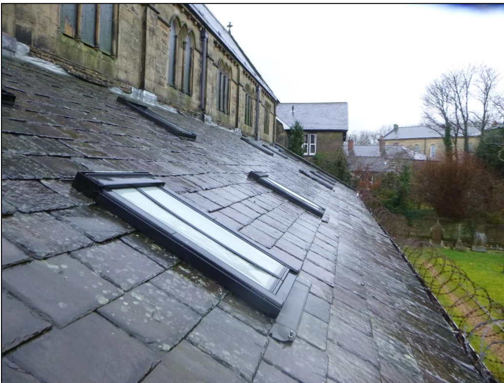
Fig.18 - Rooflights to the North Aisle
