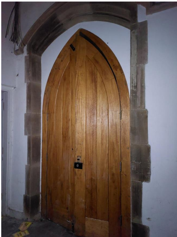
Fig.26 - Existing entrance door off Entrance Hall
