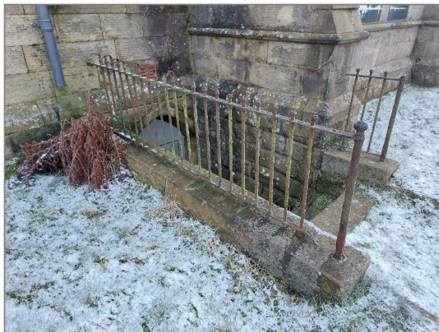
Fig.21 – Existing railings leading to crypt
