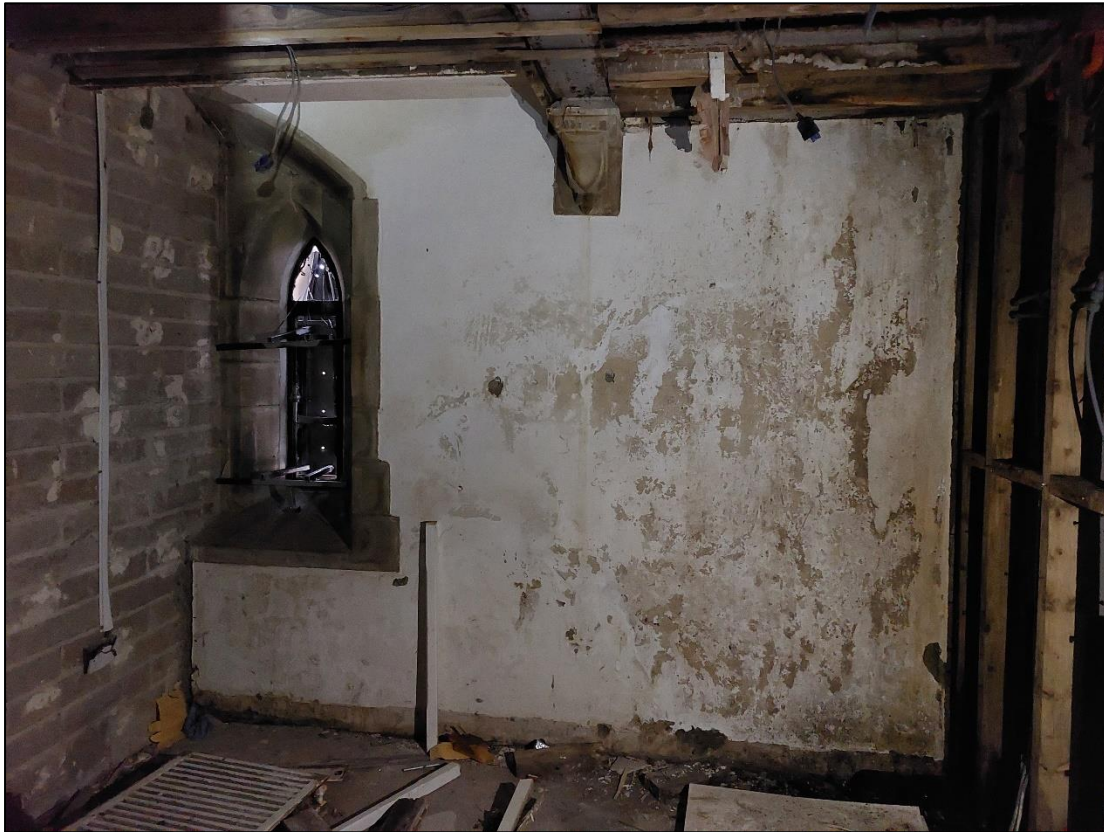
Fig.11 – Retained stone details to window and corbel.
