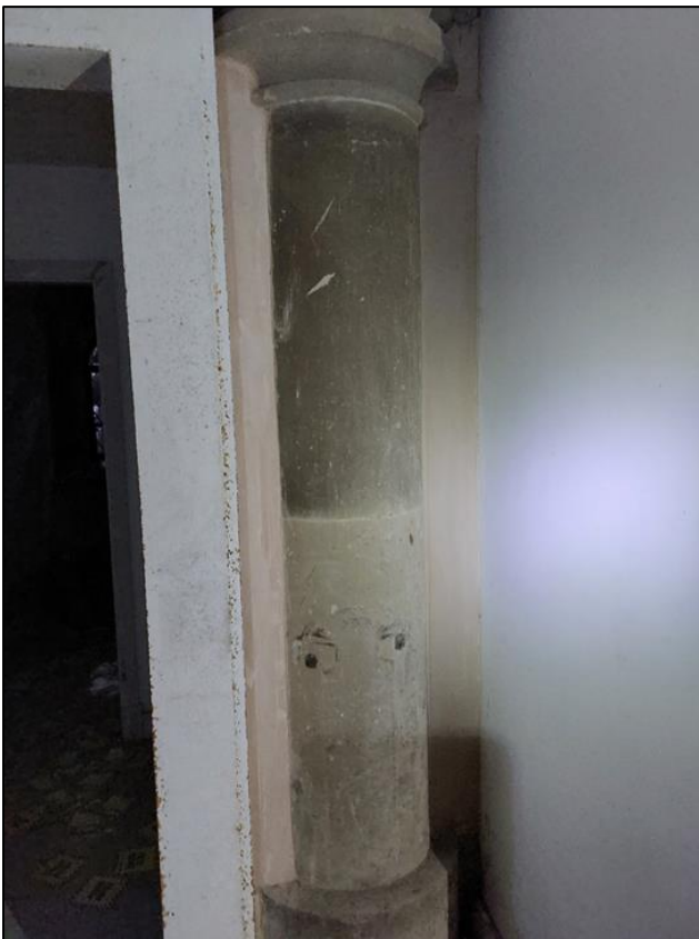
Fig.4 – Stone column No. 6 in House 4
