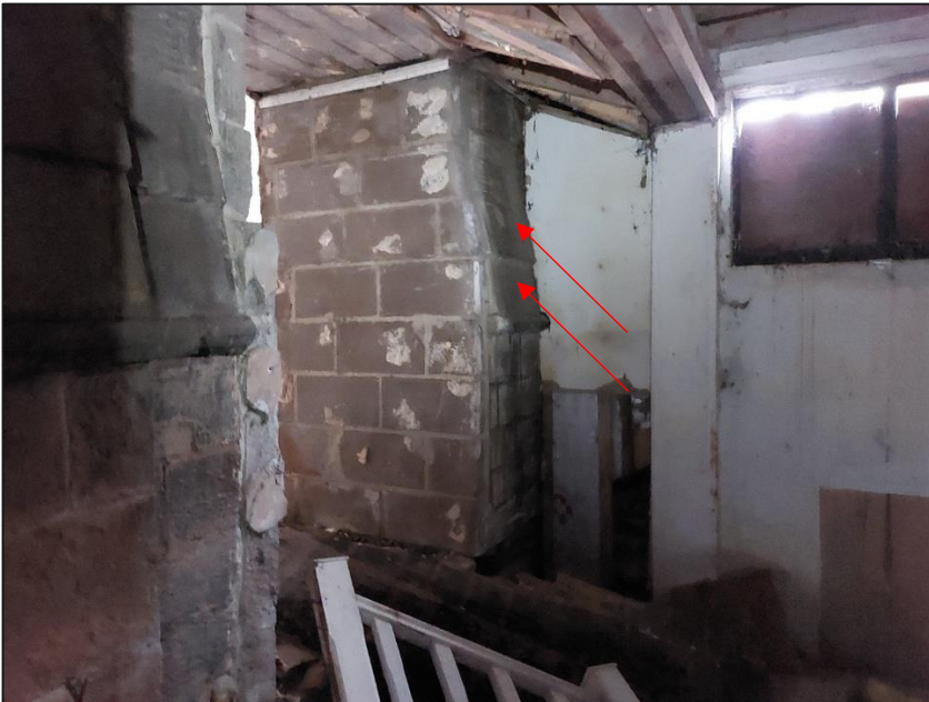
Fig.20- View of opening from first floor dormer
