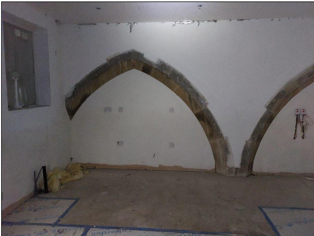
Fig.12 – Retained stone details to window and corbel.
