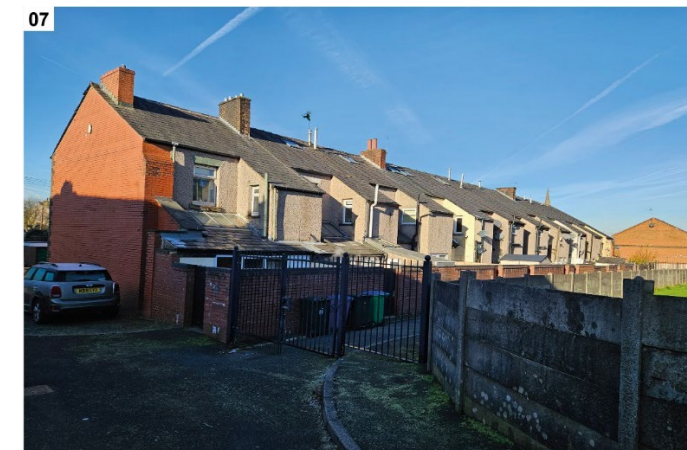
View of existing metal railings that secure the alley to the rear of the site.
