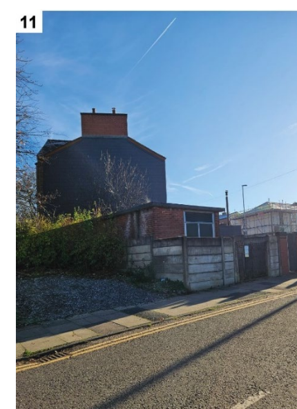
View looking towards 35 King Street.
