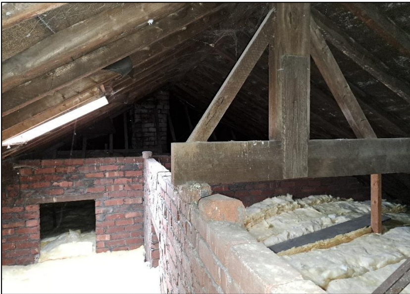
Photograph 8 showing a section of the roof void
