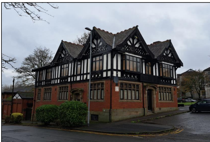
Photograph 1 showing the exterior of the building
