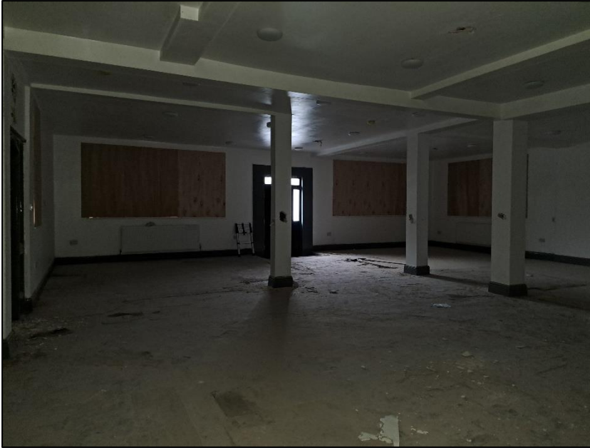
Photograph 7 showing a section of the ground floor space
