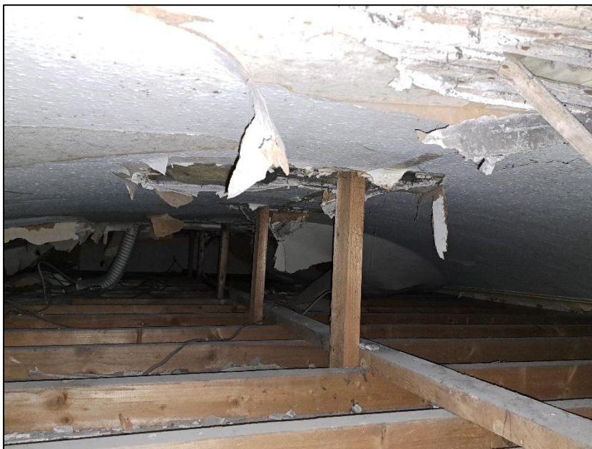
Photograph 10 showing a small roof space
