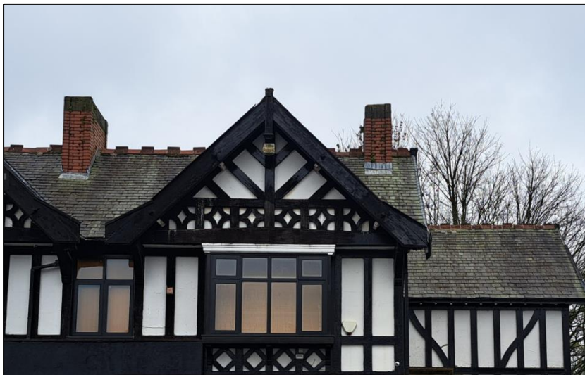
Photograph 4 showing the roof
