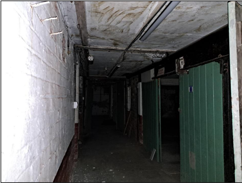
Photograph 11 showing the cellar space
