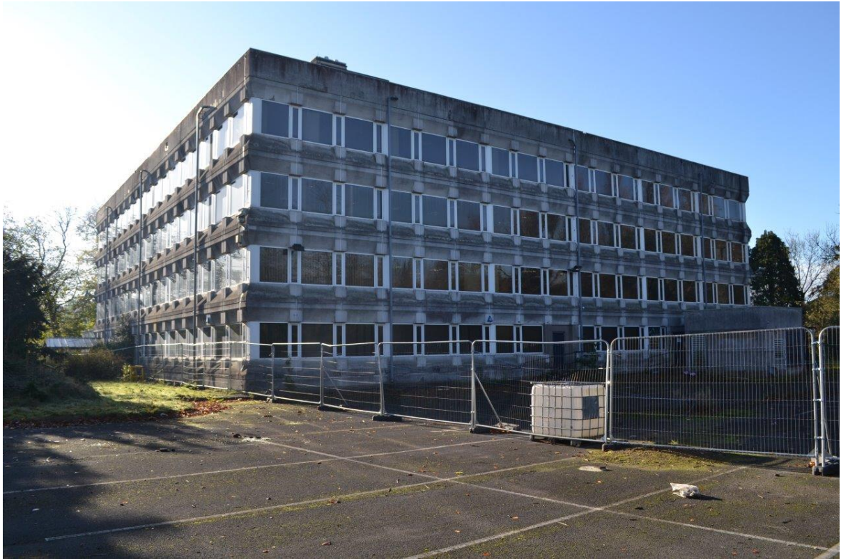
Plate 3: Sightline to the south-west towards the east-facing and north-facing elevations of Parkfield House highlighting the car parking areas laid to hardstanding.
