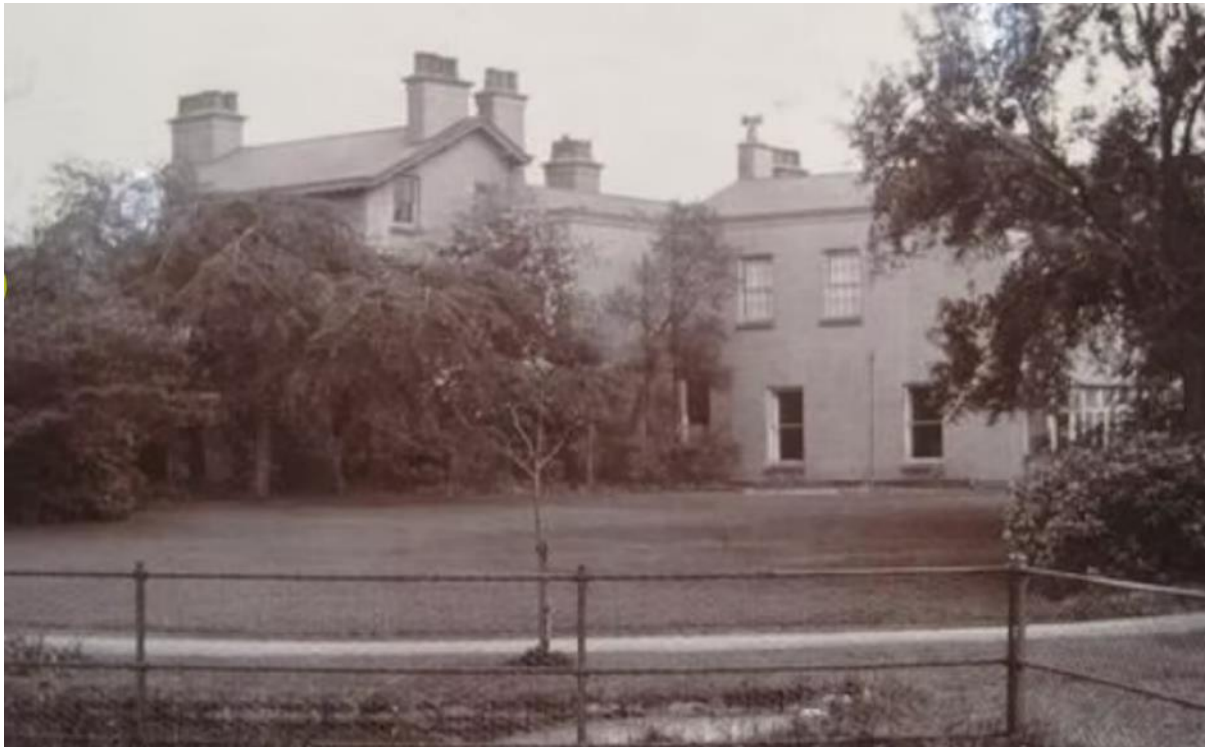
North-facing elevation of Park Field House
