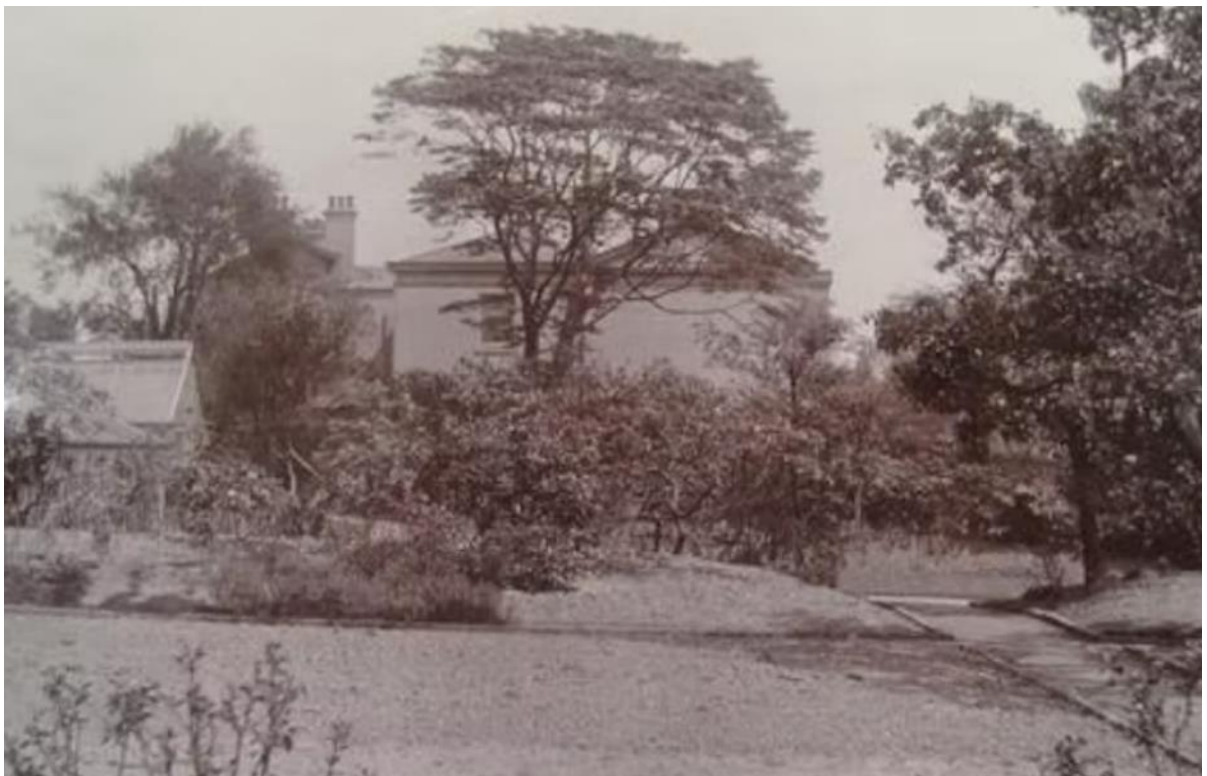
West-facing elevation of Park Field House from the gardens
