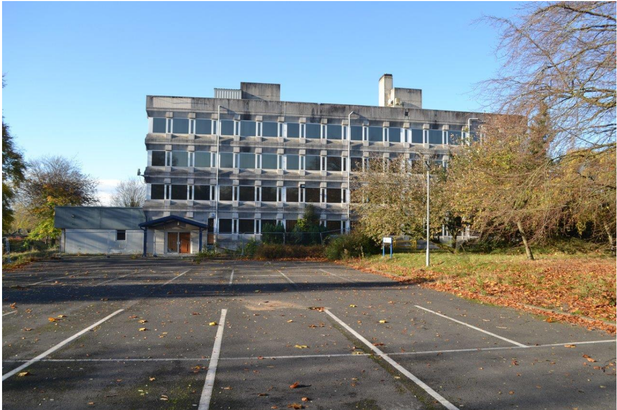
Plate 1: Sightline to the west showing the car parking area laid to hardstanding in front of the east-facing elevation of Parkfield House
