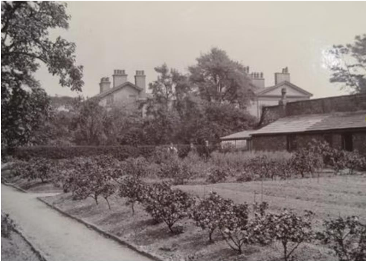
West-facing elevations of Park Field House form the walled gardens, also shows a greenhouse and lean-to utility buildings built against the garden wall
