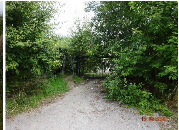
Pic 3 shows the view looking north from the junction of Cowm Top Lane and Cripple Gate Lane and showing the gate and 'A' frame intended to prevent unauthorised use of motor vehicles.
