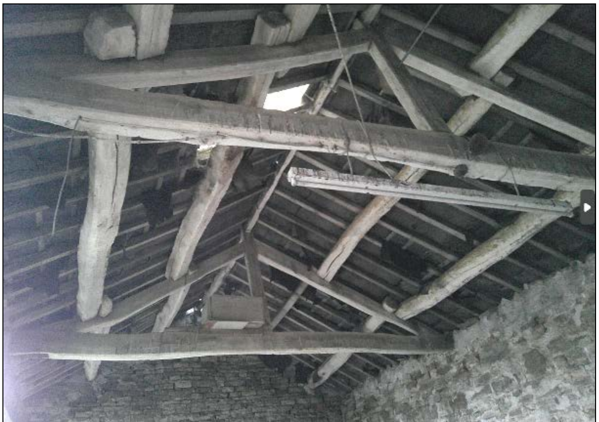
8. Its kingpost roof trusses
