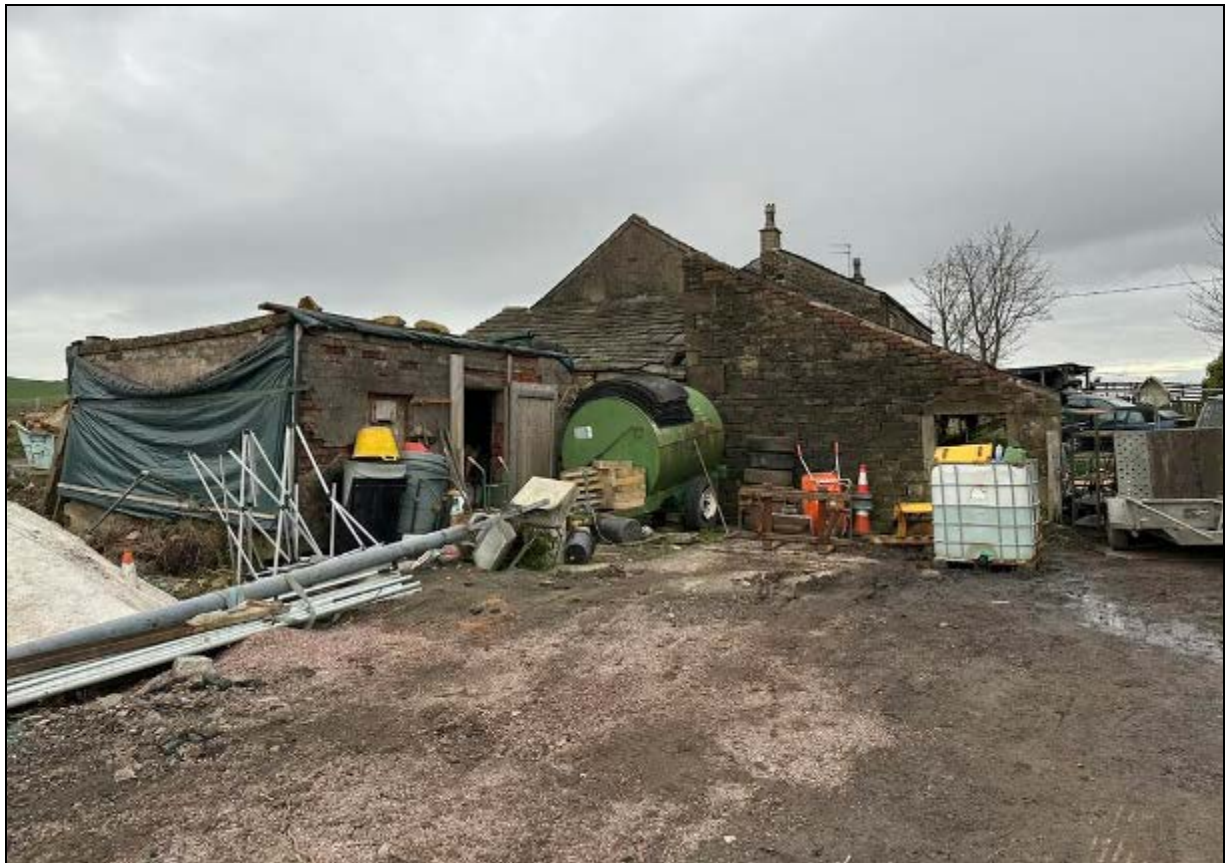
3. The barn and its additions, viewed from south
