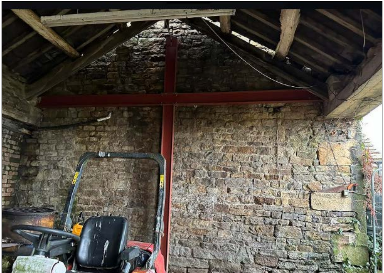
5. End wall of the house is watershot, indicating the barn is an addition
