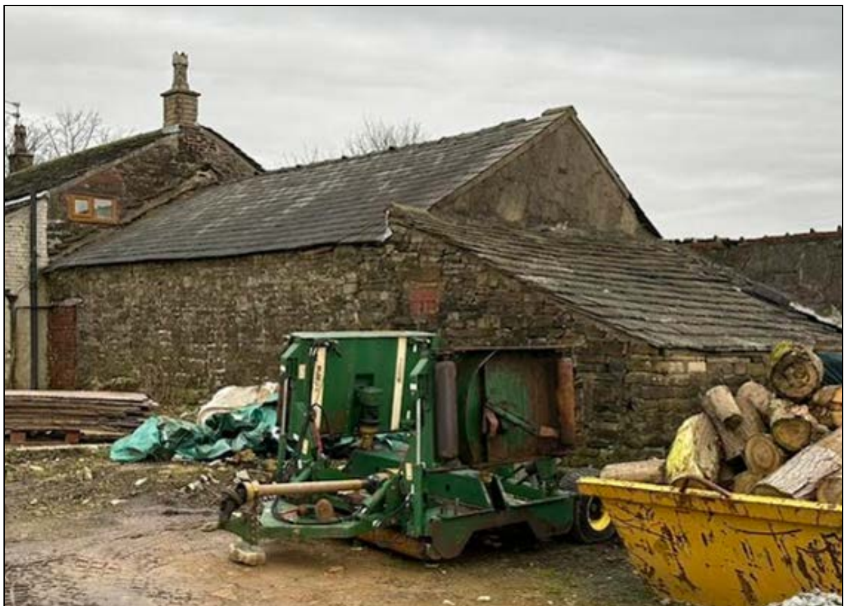
4. The barn and the outshut added at its south end
