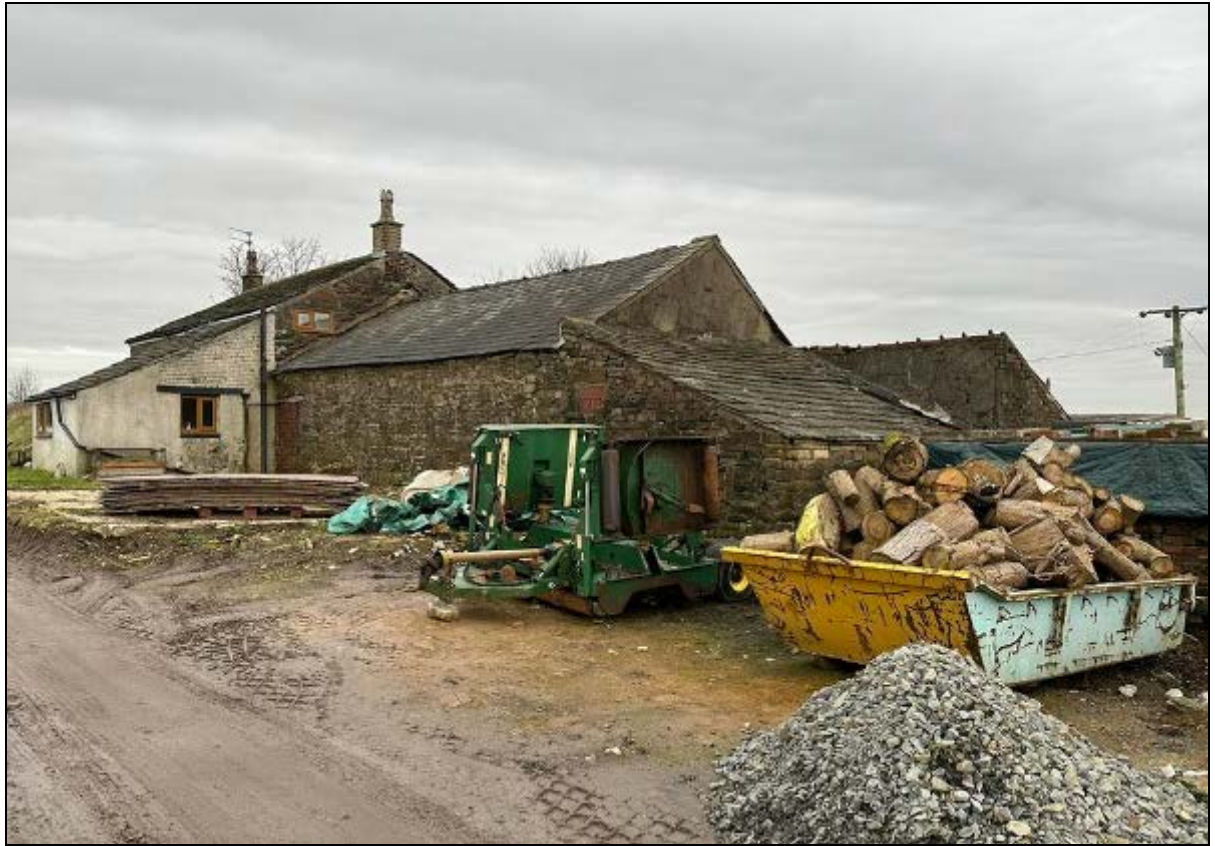
1. The barn, with farmhouse beyond
