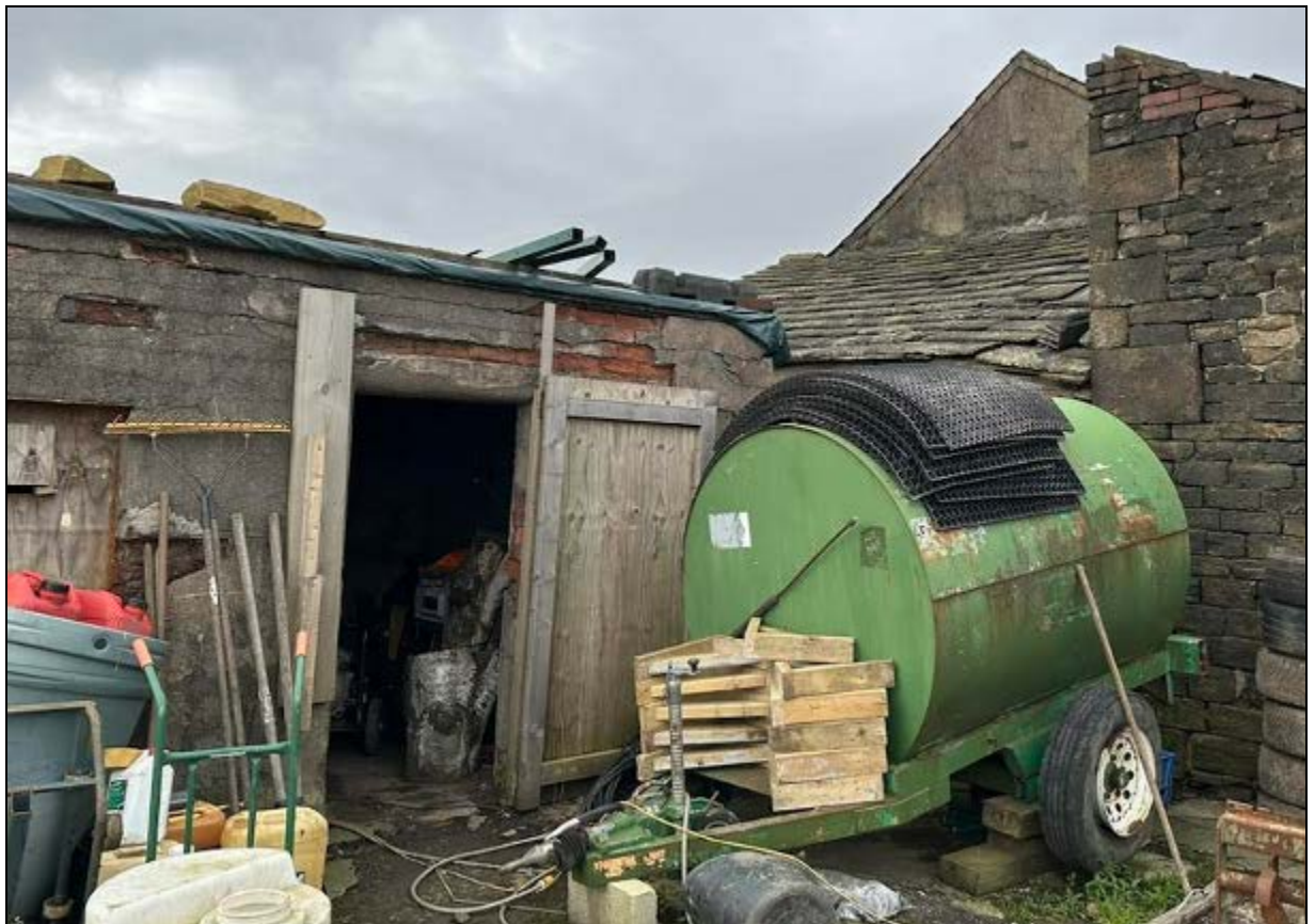
12. The early 20 th century brick outbuilding
