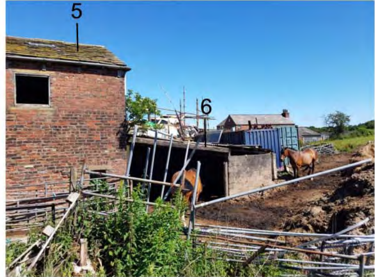
view looking northeast (rear of building 5)
