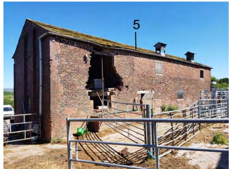
view looking northeast (rear of building 5)
