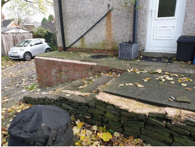
Photo 2: Repairs to edge of steps
