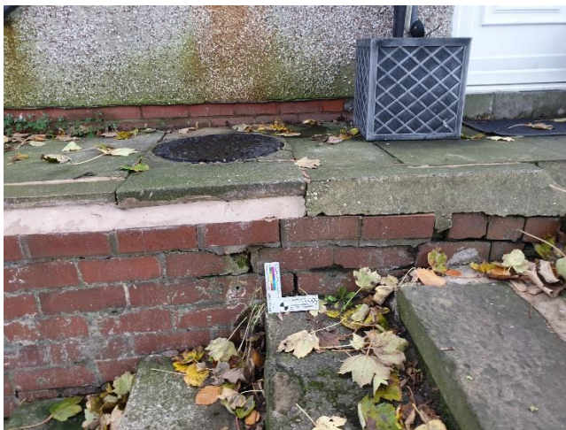
Photo 4: Repairs to brickwork adjacent to drain
