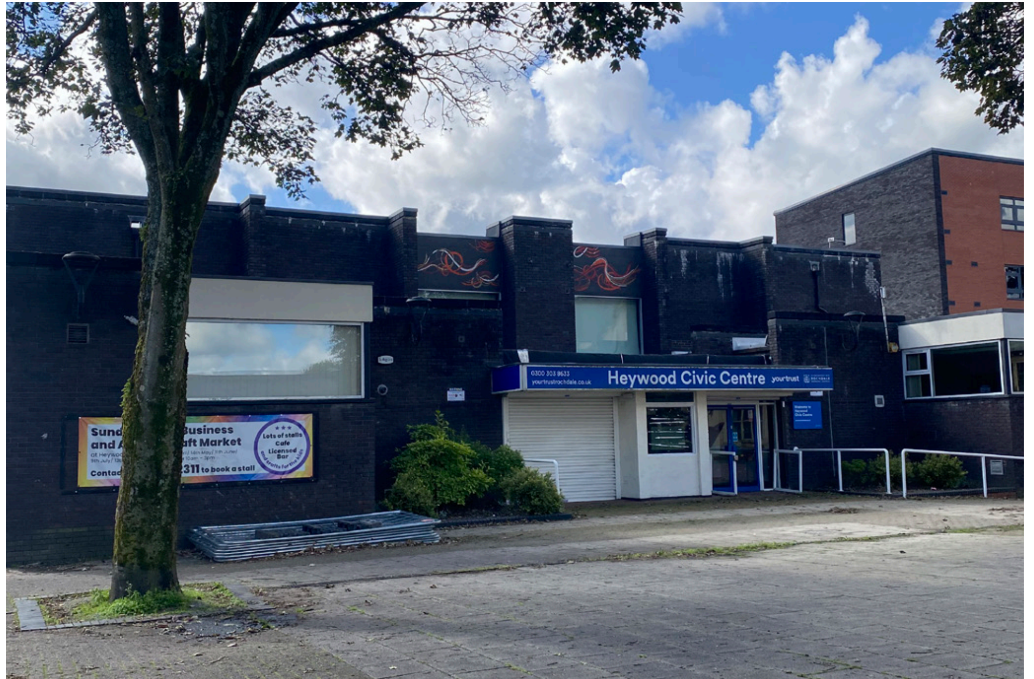
Current entrance to Heywood Civic Centre
