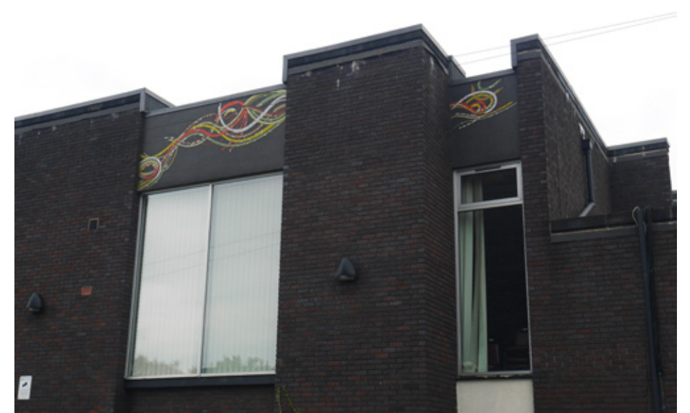
Existing View of Mosaiced Spandrel Panels
