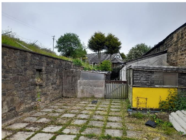
View of the rear of the property
