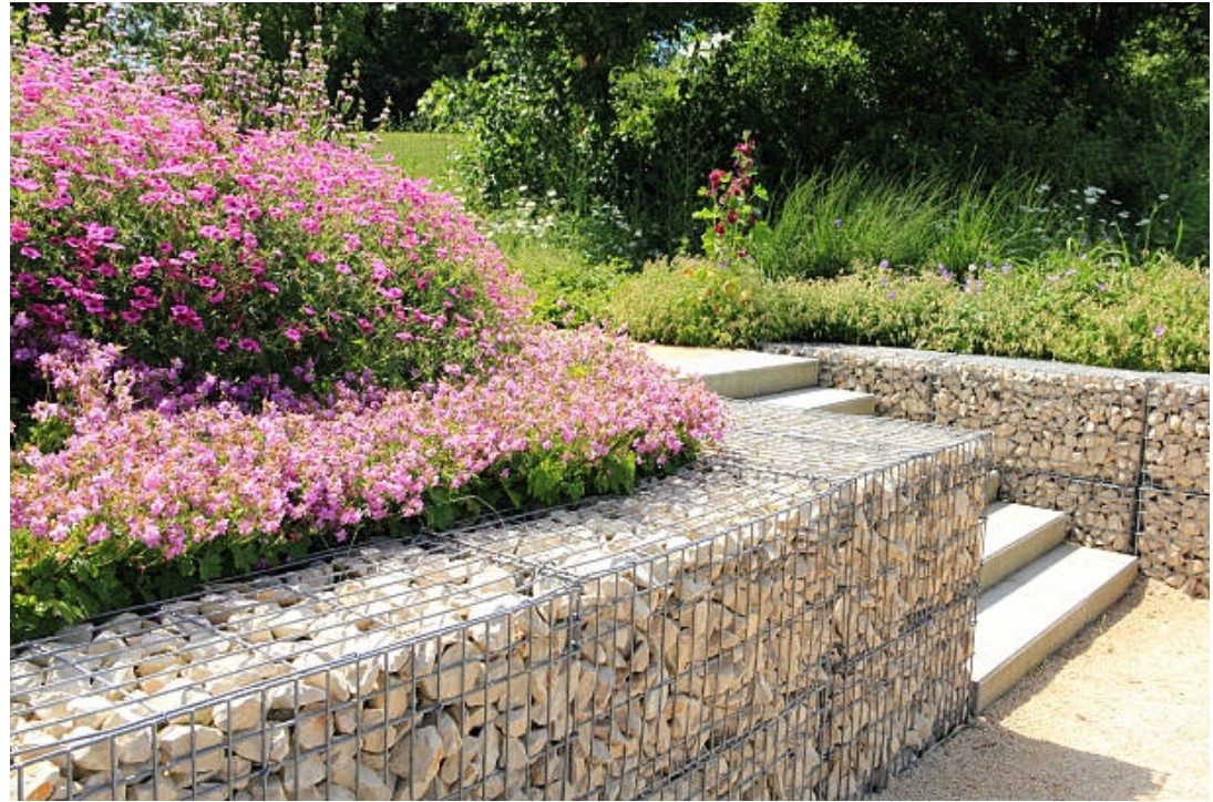
1M high gabion basket retaining walls
