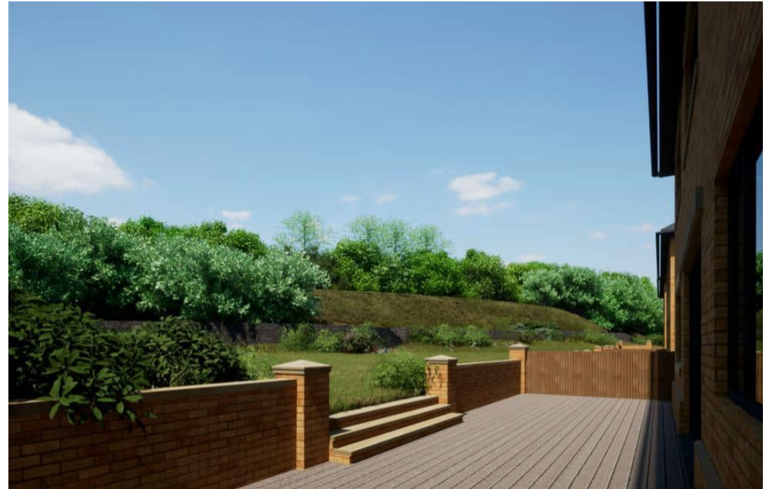
Patio and garden walls in facing bricks with stone copings to match the houses.
