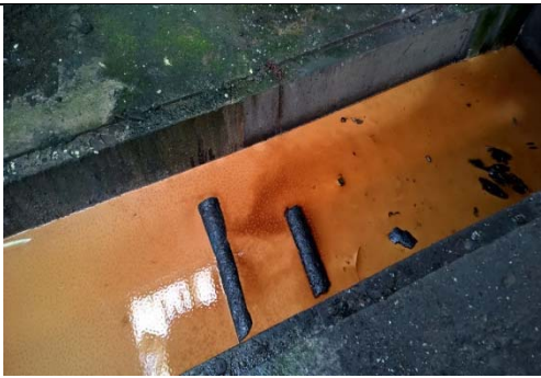
Photograph 8 (P8) Sumps with hydraulic oil were noted in former hydraulic press area.
