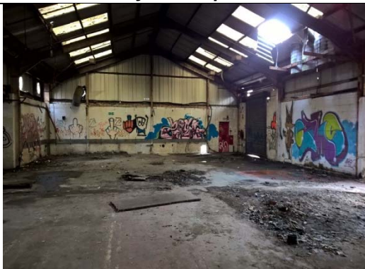
Photograph 11 (P11) Only small areas of the former Works building were safe to access.
