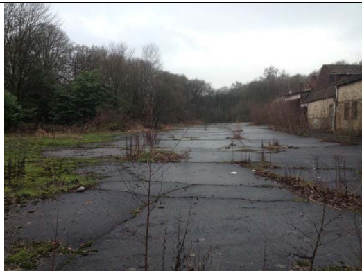
Photograph 1 (P1) Concrete yard in the south of the site.
