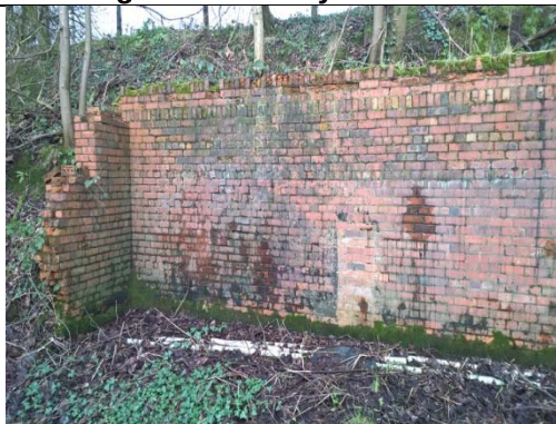
Photograph 12 (P12) Retaining wall in the north and possible former tank location.
