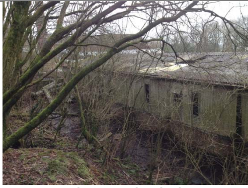
Photograph 5 (P5) Area immediately to the north of the buildings showing waterlogging.
