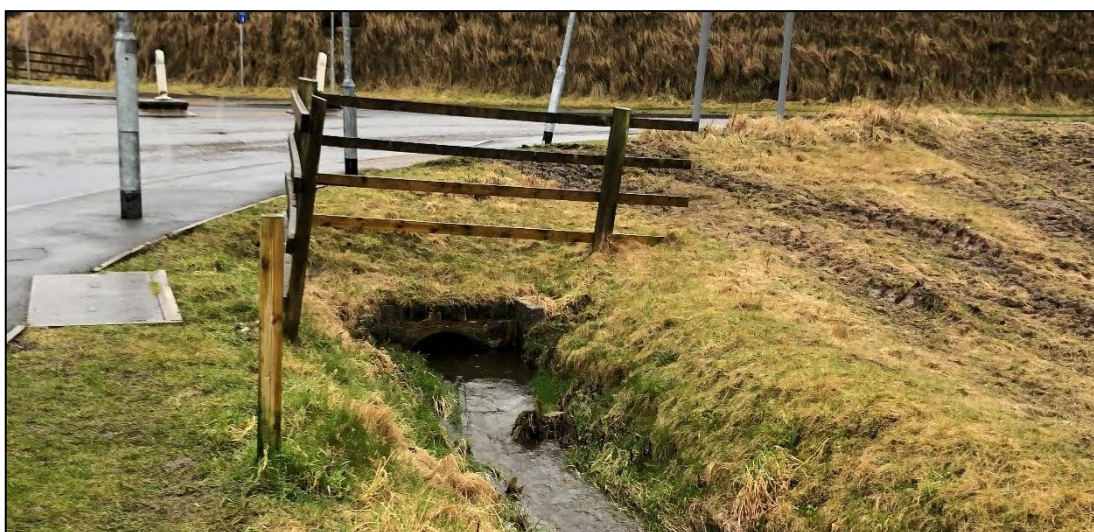
Figure 3.4: Photo taken on downstream end of circular culvert upstream of site, along the eastern boundary. (Photo taken on 10/03/21)
