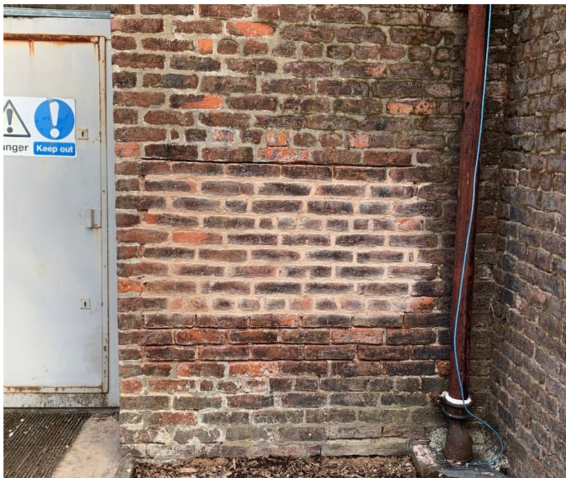
Figure.4 Lime mortar sample.
