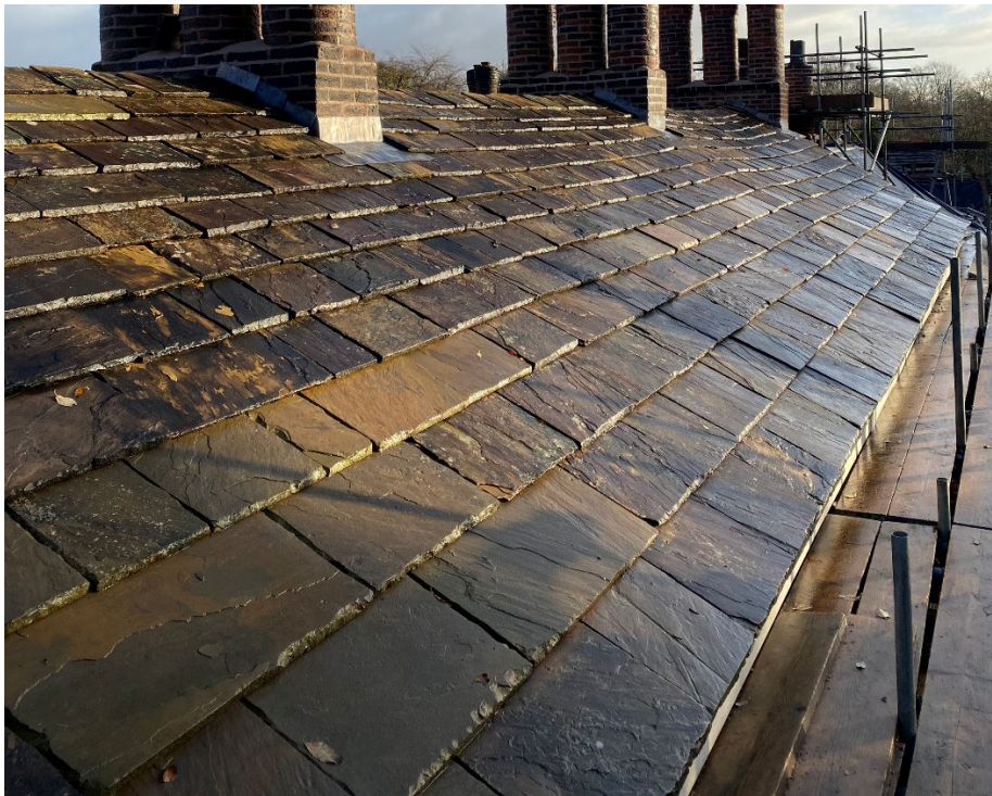
Figure. 1 Existing stone slate mixed with new slates to match existing.
