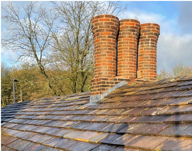
Figure.3 Brick repairs to chimneys using a mixture of existing bricks and new bricks to match existing.
