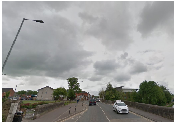
View of site from bridge over canal
