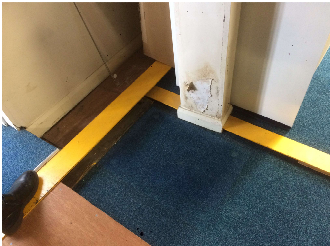
Structural Steel Insertions to Improve Roof Support
