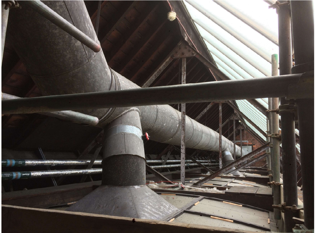
Roof Over Rear Part of Library
