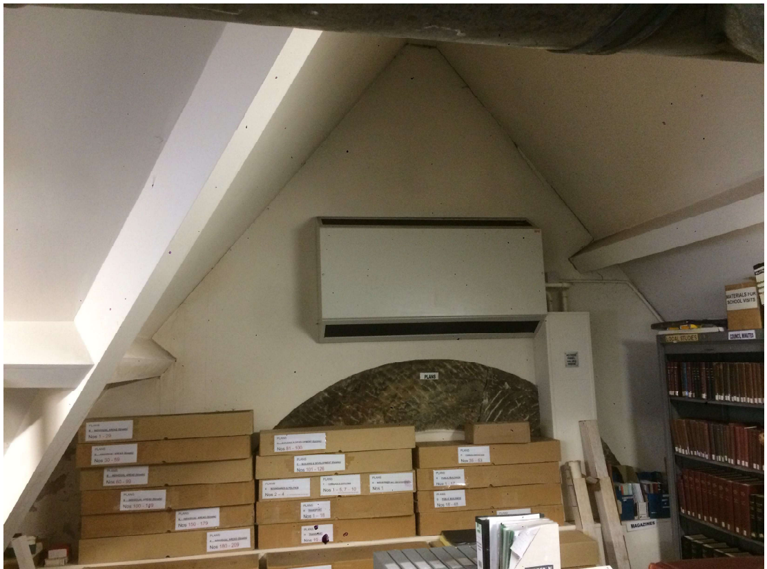
Front Right Roof Space
