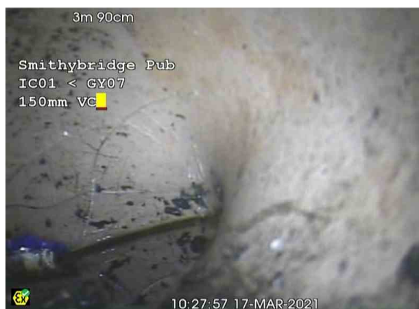
GY07X_e3f78160-28ca-4f6f-a6d9-405d2d6ae78b_20210326_102037_491.jpg, 00:00:34, 3.90 m Finish node, gully, reference: GY07
