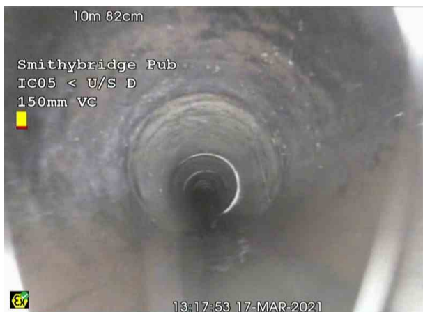
IC05 U_S DX_c32dc713-5af0-48bc-b8d8-bc4c29819c20_20210326_123 855_123.jpg, 00:01:02, 10.82 m General photograph taken at this point
