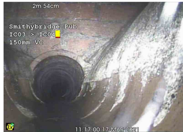
IC03X_83f4e0ee-2fd8-4424-a37d-eea1e018da35_20210326_1 12836_659.jpg, 00:00:27, 2.54 m Finish node, inspection chamber, reference: IC04
