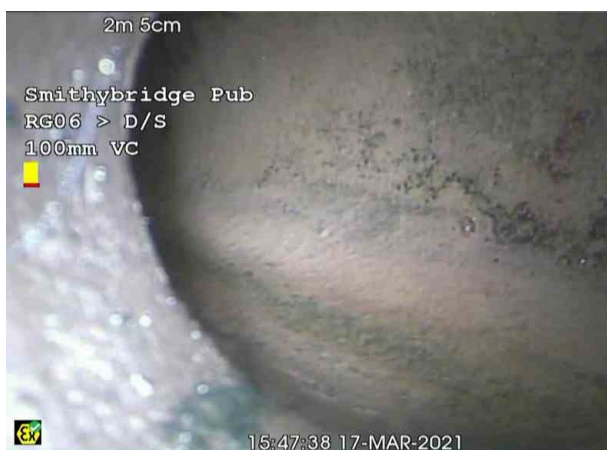
RG06X_436b3aa2-f32a-4cce-894b-458d5eec30bc_20210326_141307_109.jpg, 00:01:09, 2.05 m Finish node, other special chamber, reference: RG06 D/S, T Junction
