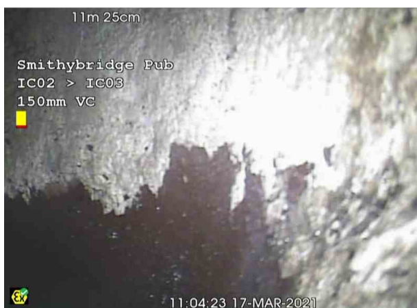
IC02X_0d4c0fe4-c70e-42f3-b07d-fe43837d78ff_20210326_11 2617_823.jpg, 00:01:16, 11.25 m Finish node, inspection chamber, reference: IC03
