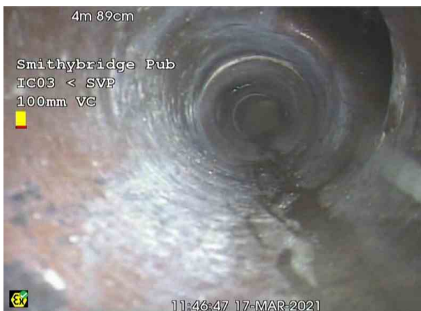
SVPX_b0ebe08b-677f-423d-9e63-7cb37e57115c_20210326_120450_924.jpg, 00:00:33, 4.89 m Junction at 2 o'clock, diameter: 100mm
