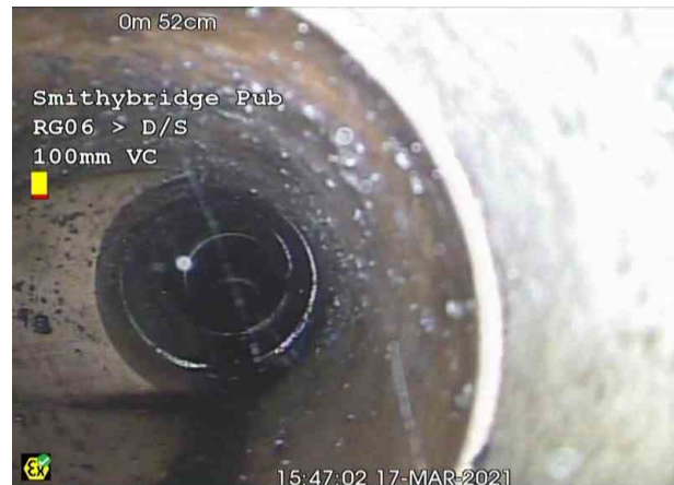
RG06X_3700d764-5051-4fc4-9839-647e2de48980_20210326_141104_473.jpg, 00:00:33, 0.52 m Junction at 9 o'clock, diameter: 100mm
