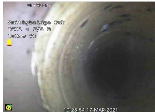
IC01 U_S BX_d01a7057-fa8b-4ee8-9392-acd33942c42b_20210326_103 016_752.jpg, 00:00:12, 0.93 m Point repair, localised lining from 12 o'clock to 12 o'clock, start
