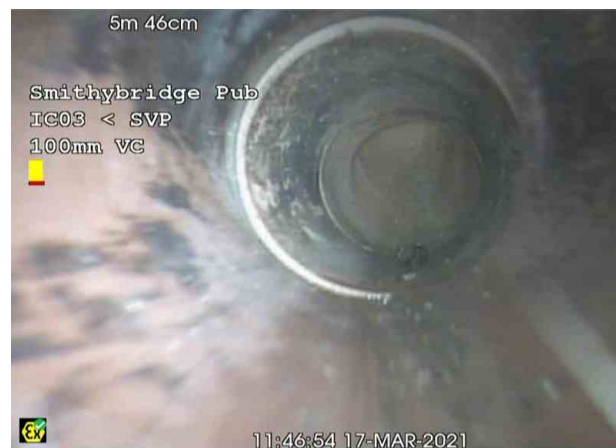
SVPX_62bcf494-8c00-4155-80bc-5146b88080fe_20210326_120527_157.jpg, 00:00:40, 5.46 m General photograph taken at this point
