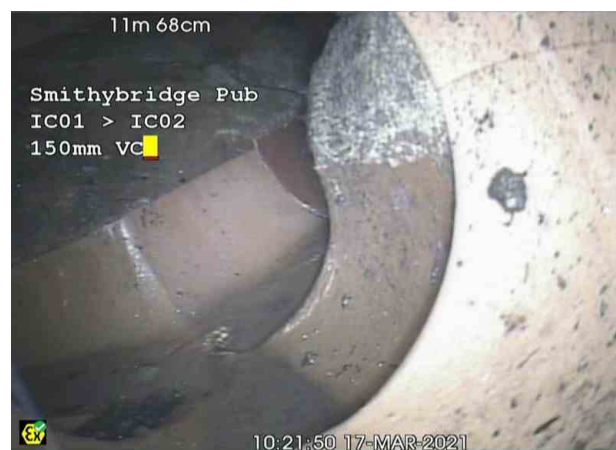
IC01X_fae65e3b-d66d-42b9-bde6-6874127e1edd_20210326_101607_541.jpg, 00:01:15, 11.68 m Finish node, inspection chamber, reference: IC02
