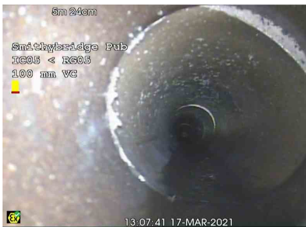
RG05X_3cc1f169-8a7e-4505-a0a4-dda083e1e434_20210326_121353_520.jpg, 00:00:31, 5.24 m General photograph taken at this point
