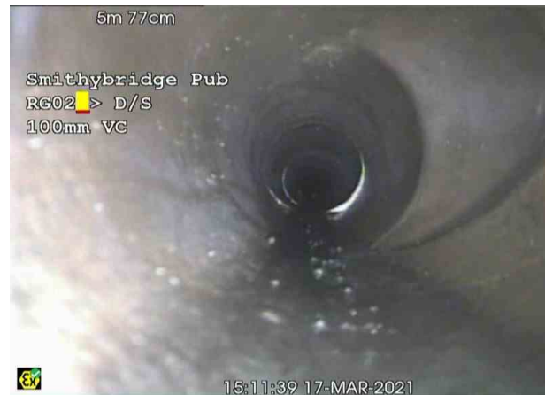
RG02X_67cb7ecb-5983-4ab8-9259-0fe1dee003fe_20210326_135053_042.jpg, 00:01:55, 5.77 m General photograph taken at this point
