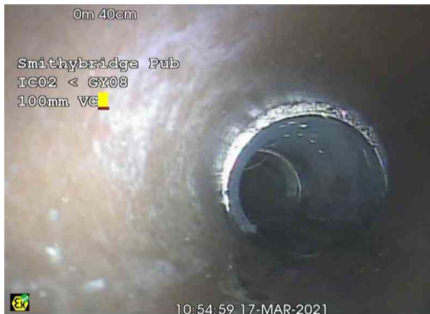
GY08X_eb75e575-9715-4534-94f6-f420e8364a0b_20210326_105238_660.jpg, 00:00:00, 0.40 m General photograph taken at this point
