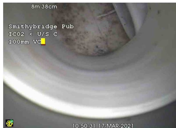
IC02 U_S CX_02fdb13b-785b-42cd-8000-b0512d5cf0cf_20210326_1001 42_734.jpg, 00:00:54, 8.38 m Finish node, other special chamber, reference: IC02 U/S C, Waste discharge point
