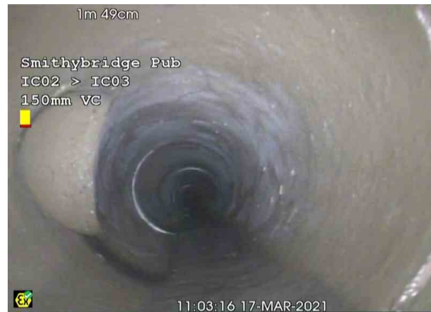
IC02X_364c3182-ee9f-4bfb-a9cb-aff01ec17db7_20210326_112159_505.jpg, 00:00:10, 1.49 m Junction at 10 o'clock, diameter: 100mm
