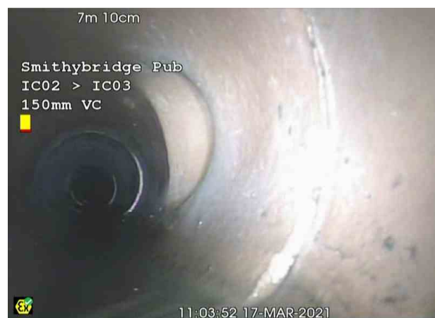
IC02X_6c7172f1-f529-4103-9b40-56763bc648ec_20210326_112416_943.jpg, 00:00:46, 7.10 m Junction at 2 o'clock, diameter: 100mm
