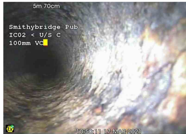
IC02 U_S CX_f40f73d4-74ac-47b8-8c70-8ca3797d4c23_20210326_0956 17_417.jpg, 00:00:34, 5.70 m General photograph taken at this point
