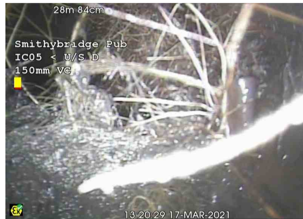
IC05 U_S DX_e148923e-c4e2-4c17-84b8-2d7ced156081_20210326_124 425_674.jpg, 00:03:39, 28.84 m Finish node, inspection chamber, reference: IC05 U/S D, Buried / Shown as IC05 on the screen
