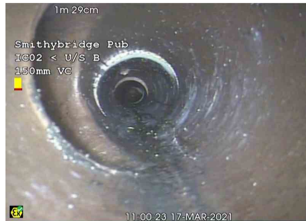
IC02 U_S BX_835b8aab-5741-41e1-9aac-735842a1afe5_20210326_110 753_842.jpg, 00:00:07, 1.29 m Junction at 8 o'clock, diameter: 150mm
