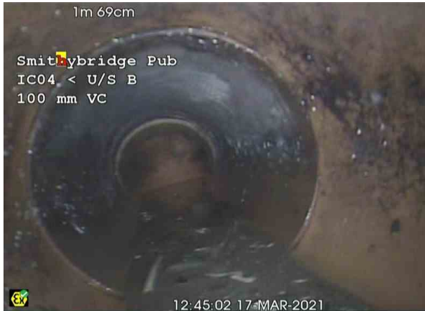
IC04 U_S BX_3a19d02f-3985-415d-a1de-1ce7cee48966_20210326_120 949_034.jpg, 00:00:17, 1.69 m General photograph taken at this point
