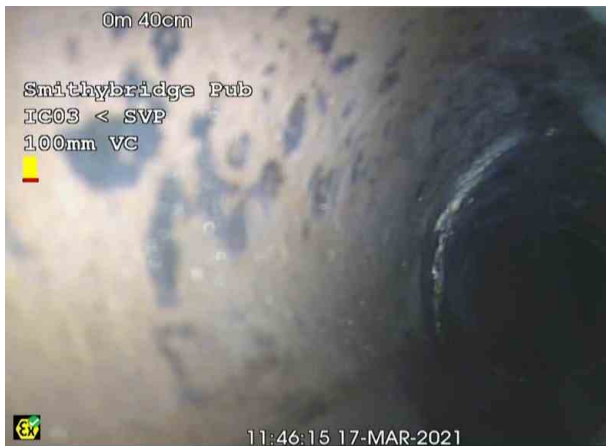
SVPX_fe868a87-72a2-4fac-9739-69fe3592c8f4_20210326_115701_230.jpg, 00:00:00, 0.40 m General photograph taken at this point
