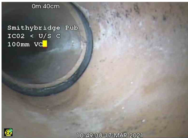
IC02 U_S CX_c05dca78-e744-4819-b1ed-a5d5036f9838_20210326_095 130_462.jpg, 00:00:00, 0.40 m General photograph taken at this point
