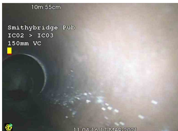
IC02X_649e419c-124c-4f1e-8107-f98a7563e25f_20210326_1 12551_197.jpg, 00:01:10, 10.55 m General photograph taken at this point
