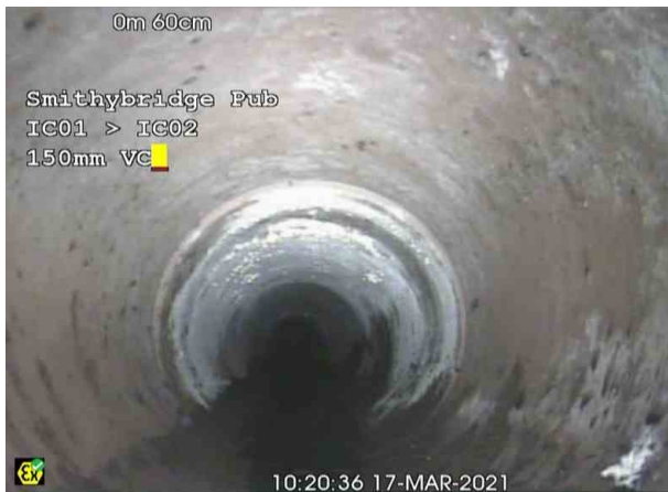
IC01X_bffedaaf-4910-402c-99f7-d0e334cd5fe1_20210326_100658_049.jpg, 00:00:01, 0.60 m General photograph taken at this point
