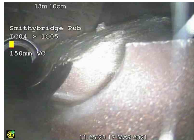
IC04X_3caafd62-505b-45ff-9d04-3c207b800e15_20210326_1 13409_657.jpg, 00:01:35, 13.10 m Finish node, inspection chamber, reference: IC05
