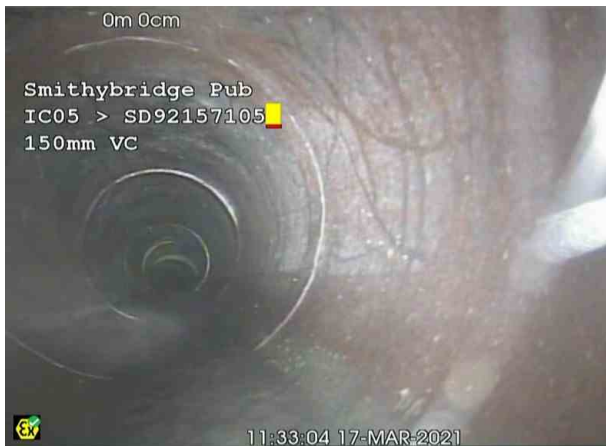
IC05X_829f2e07-1144-4736-ba59-2aec8c64bc2f_20210326_1 13437_203.jpg, 00:00:00, 0.00 m General photograph taken at this point
