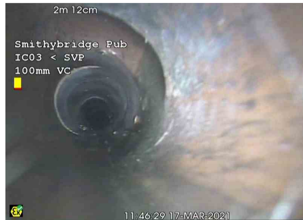
SVPX_731bb806-4714-4449-ae77-cf0db3dc7702_20210326_120422_045.jpg, 00:00:15, 2.12 m Junction at 2 o'clock, diameter: 100mm
