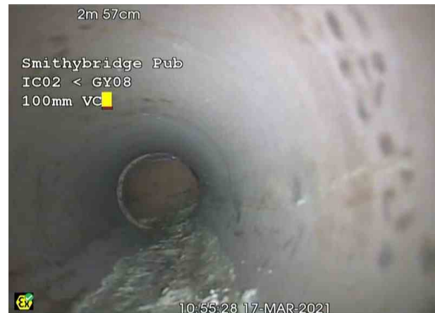
GY08X_da1f80c1-b3d6-40e5-8a65-42b870347a63_20210326_110109_422.jpg, 00:00:30, 2.57 m General photograph taken at this point
