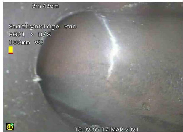
RG01X_3fbc5cbf-7d72-4847-8a92-9fedb3a477a7_20210326_134713_318.jpg, 00:01:21, 3.43 m Finish node, other special chamber, reference: RG01 D/S, T Junction
