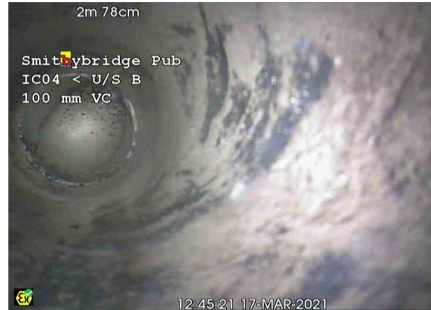
IC04 U_S BX_cbb955bb-b81c-472f-b187-6a448b6202c6_20210326_121 153_173.jpg, 00:00:37, 2.78 m Finish node, other special chamber, reference: IC04 U/S B, Node point from building
