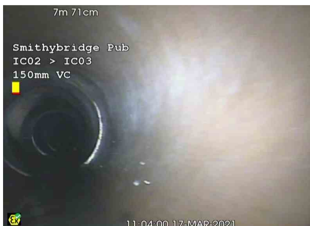
IC02X_8ddd73b6-77aa-4340-bf19-cdd7b9f01124_20210326_1 12447_119.jpg, 00:00:54, 7.71 m Junction at 10 o'clock, diameter: 100mm
