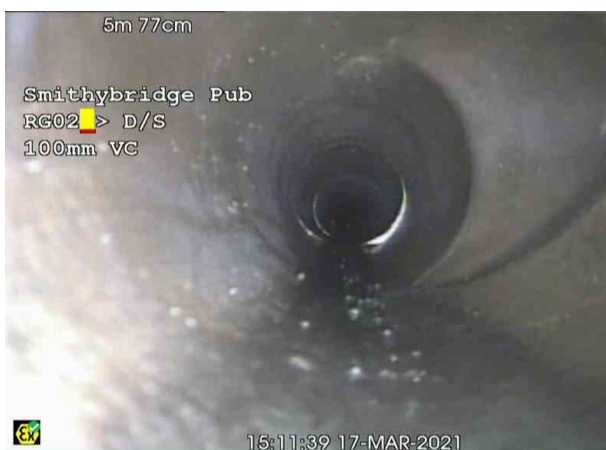
RG02X_dc1e3951-a39f-495d-9086-abf775369a2a_20210326_135107_487.jpg, 00:01:55, 5.77 m Junction at 2 o'clock, diameter: 100mm
