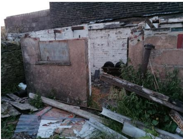
PHOTO 9 South-western Elevation of Former Extension
