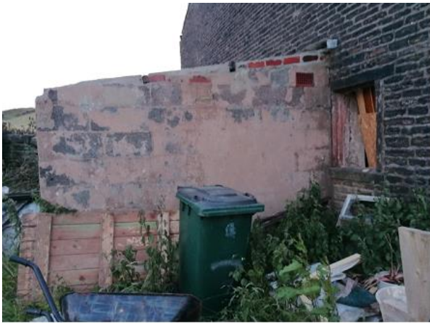
PHOTO 7 Eastern Elevation of Former Extension
