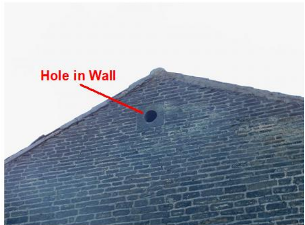
PHOTO 10 Southern Gable End
