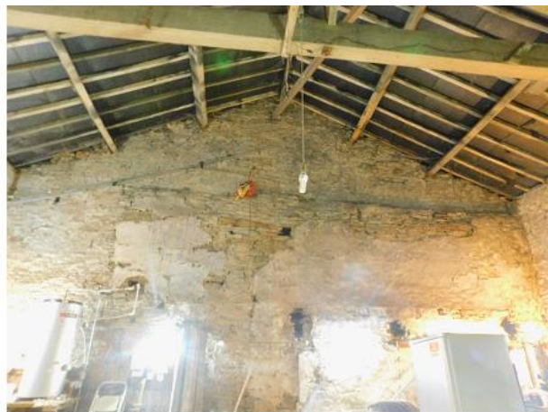
PHOTO 20 Inside View of Southern Elevation
