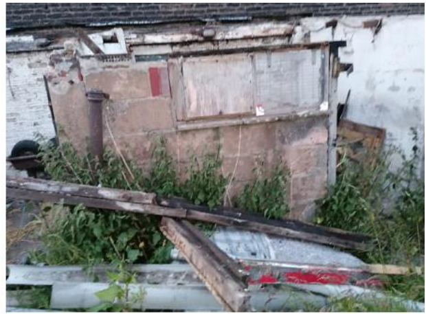
PHOTO 8 South-eastern Elevation of Former Extension
