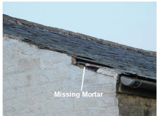
PHOTO 16 Upper North-western Corner
