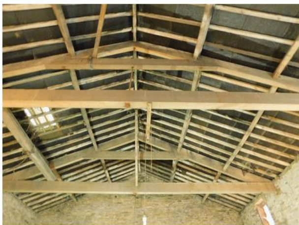
PHOTO 21 Underside of Roof
