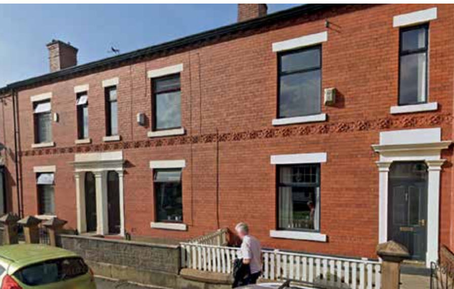
Row of Victorian terraces along Heywood Road with decorative teracotta tile detailing
