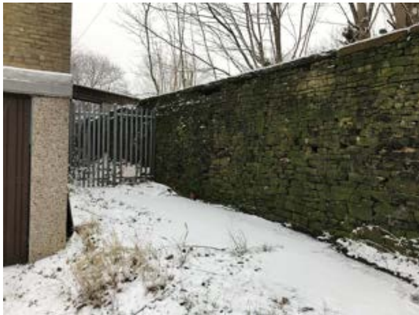
Photograph 4 – View of retaining wall which is present at the southern extent of the undeveloped area of the site.
