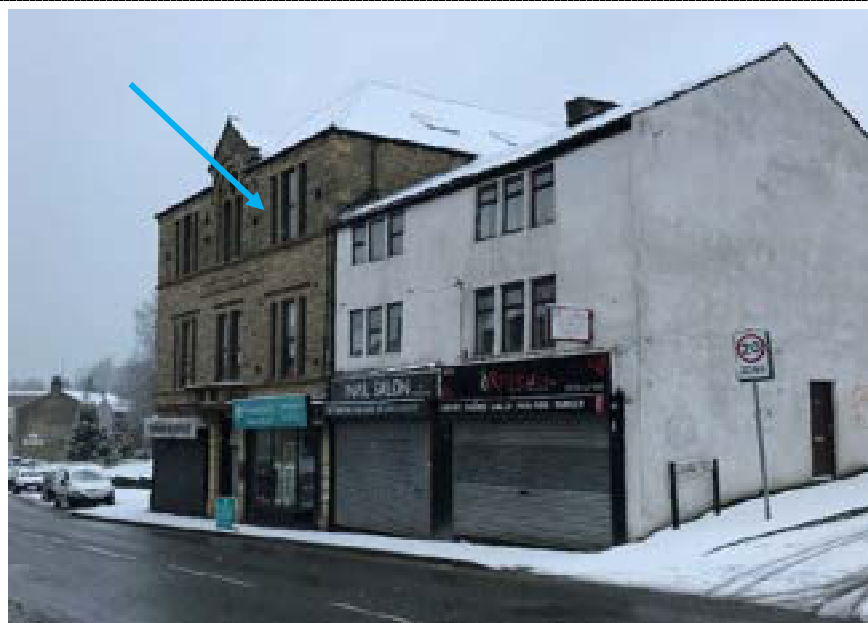
Photograph 7 – View of the the frontage of the existing building (Stone building), with retail properties shown on ground floor level. Blue arrow shows floor subject to this report.
