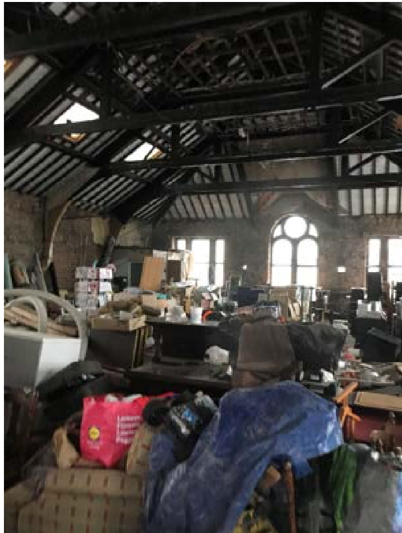
Photograph 6 – View of internal area of upper floor in the existing building which is to be converted into residential apartments.
