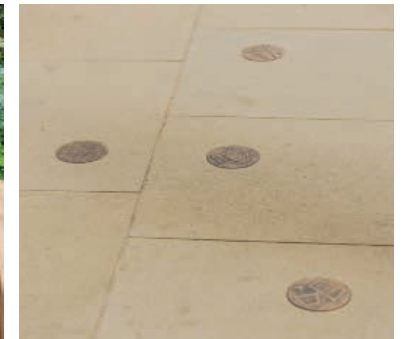
Artworks on metal studs incorporated within paving
