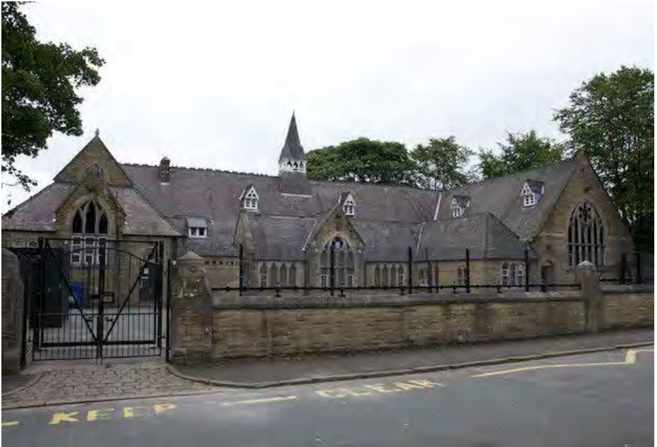
3 View of the west elevation.
