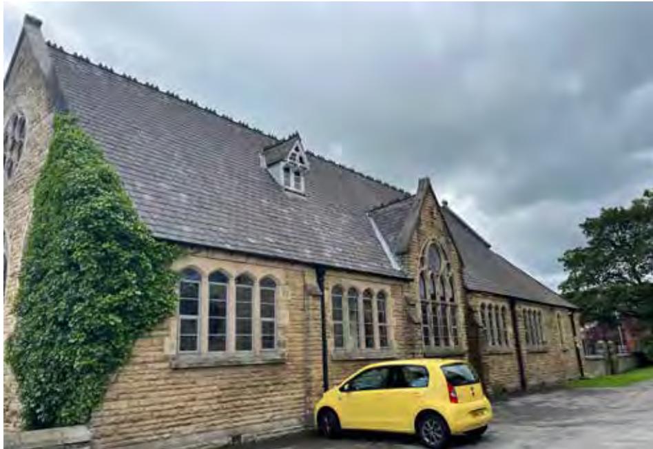
2 View looking towards the north elevation.
