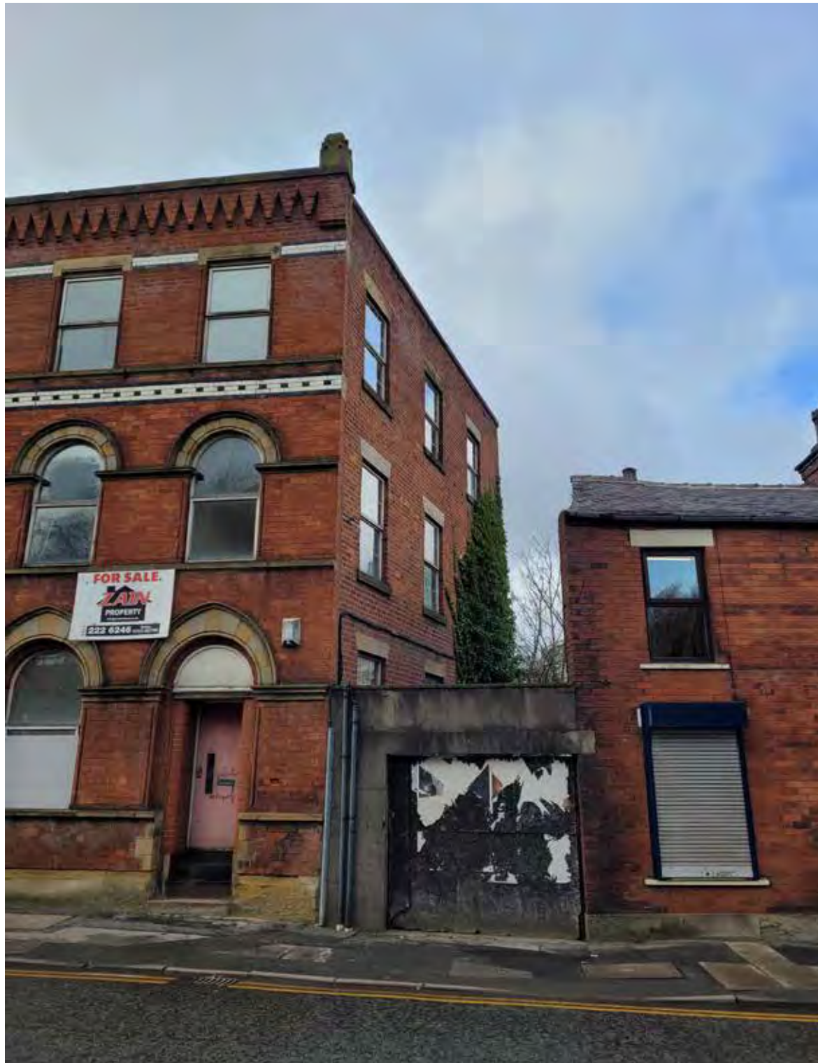
East Elevation External
