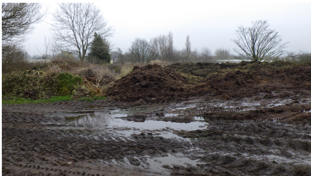
Photo 1 – Northern yard area holding stockpiles of demolition rubble, road planings and gravels
